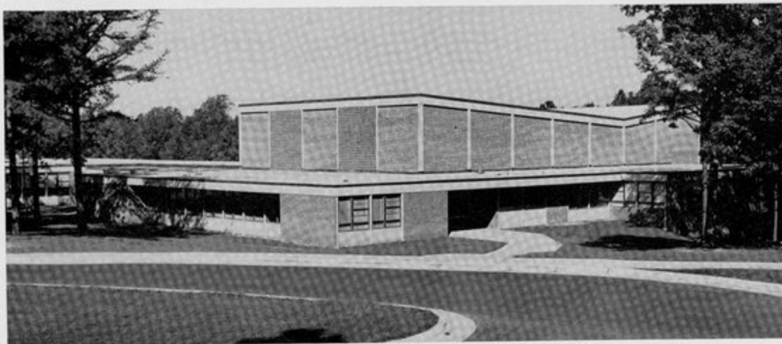
LEROY MARTIN JUNIOR HIGH SCHOOL, Raleigh, N. C. EDWARDS, McKIMMON & ETHEREDGE, Raleigh, N. C., Architects; EZRA MEIR & ASSOCIATES, Raleigh, N. C., Engineers; WILLIAM C. VICK, Raleigh, N. C., Contractor.
