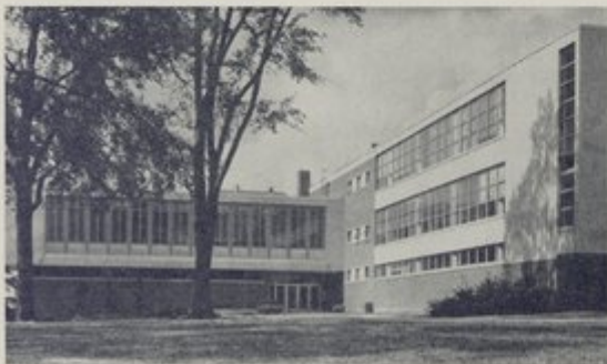
AUBURN UNIVERSITY, Auburn, Alabama — Biggin Hall, completed in August, 1951, cost, without furnishings, the sum of $434,783 and contains 51,069 sq. ft. of space. As a self-contained unit it houses activities of the School of Architecture and the Arts. Architects for the building were Pearson, Tittle and Narrows of Montgomery.
