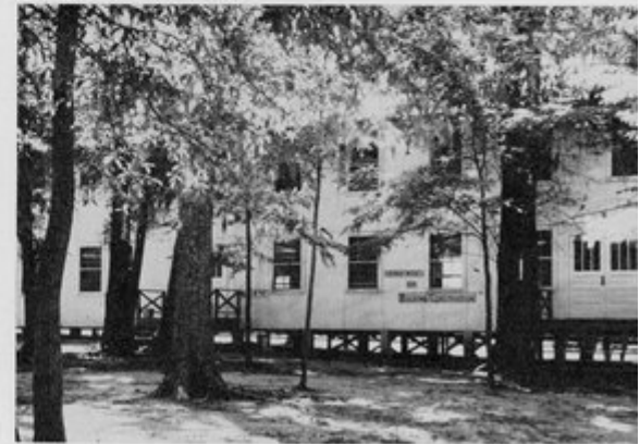
Department of Building Construction is in Building "K"—a temporary, wartime shack, but utilized since 1946.
