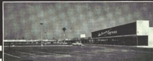
EXTERIOR VIEW OF THE NEW PALM SPRINGS SHOPPING CENTER
