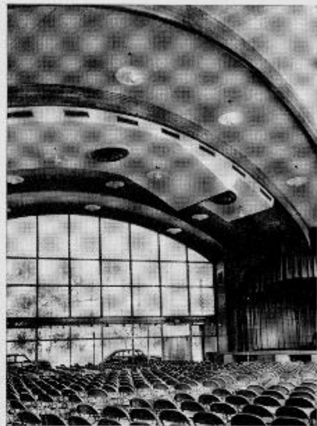
Sanford Civic Center, Sanford, Fla. Six Rilco radial arches span 84' with radius of 52'; 1 tangent arch spans 34' 2 1/4", with radius of 9' 4"; 1 pitched beam 61' in length; 94 flat beams up to 59' in length.
