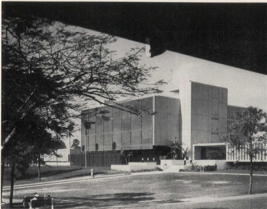
J. Neville McArthur Building, University of Miami School of Engineering.
