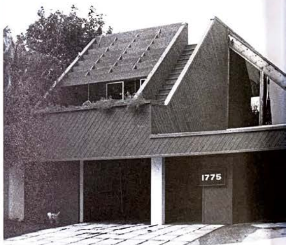
HONORABLE MENTION Addition to a Residence ARCHITECT: Daniel E. Adache
