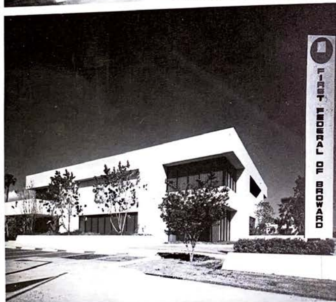
HONORABLE MENTION First Federal of Broward ARCHITECTS: William T. Vaughn & Robert J. Wunsch
