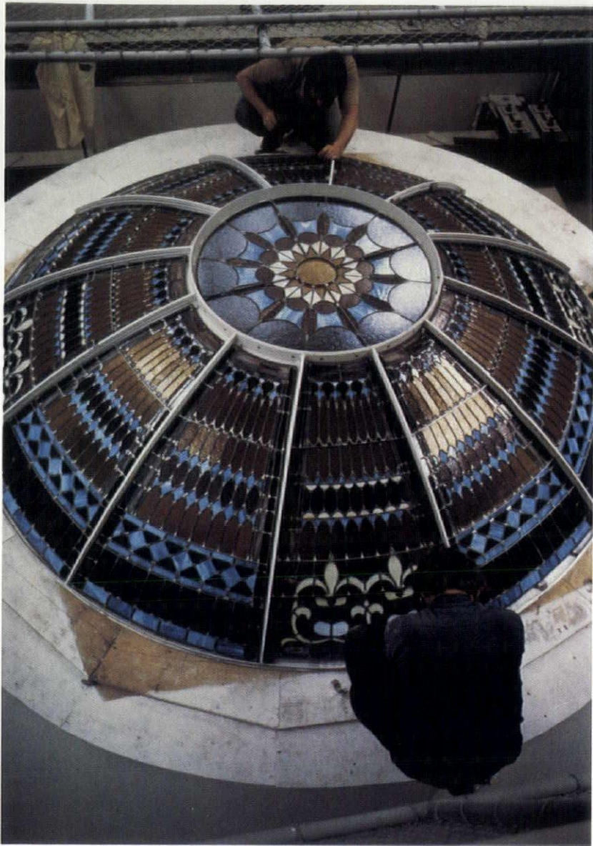
Craftsmen put the finishing touches on the artglass dome over the Capitol rotunda. The twelve panel dome contains sixteen different types of glass and 3,250 different pieces. Photo by Kenneth R. Smith, AIA.
