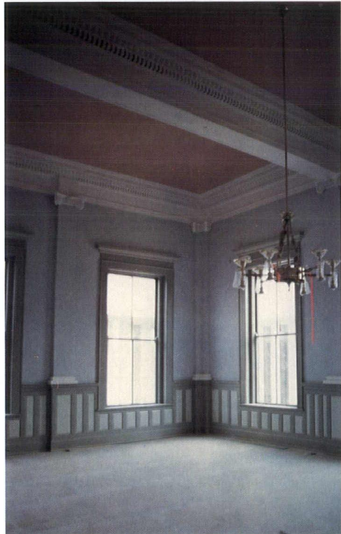
Restored House of Representatives Chamber. Note the partially laid battleship linoleum and the light fixtures which are exact reproductions of the original. Photo by Randy Atlas.
