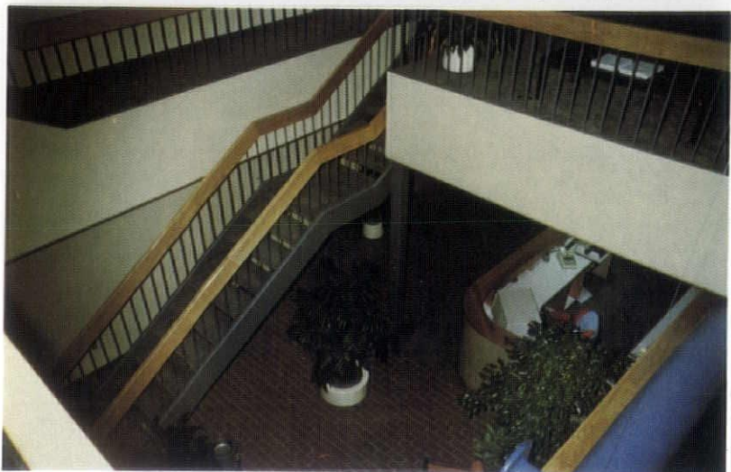
View of lobby from third floor conference room level showing mezzanine level in between. Photo by Danny Pietrodangelo.
