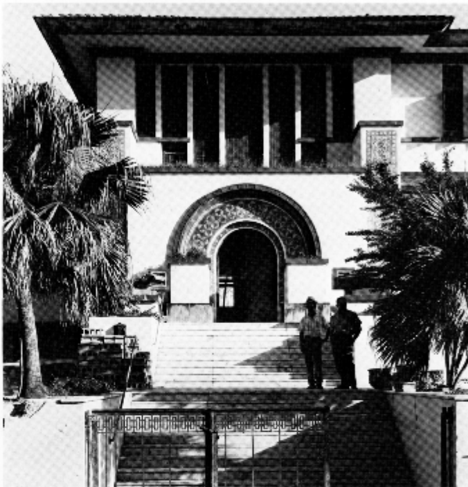
Detail of entrance to Georgetti Mansion in San Juan
