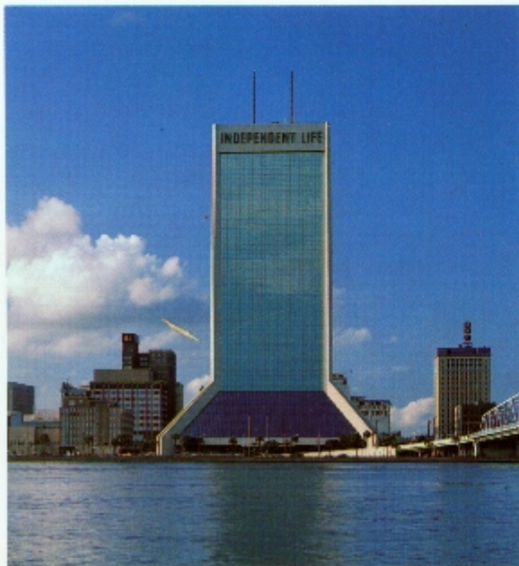
The Independent Life Building, view of south elevation from across the St. John's River Photo by Jeff Brune.
