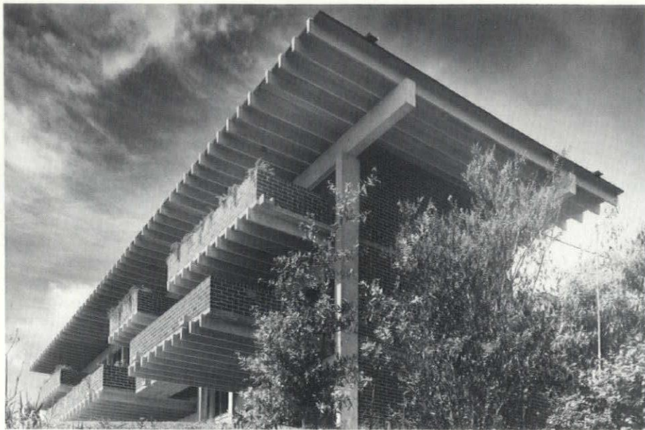
Gene Leedy's Dorman Residence built in Winter Haven in 1961 is typical of the straightforward structural expression which gives great strength to Leedy's work.
