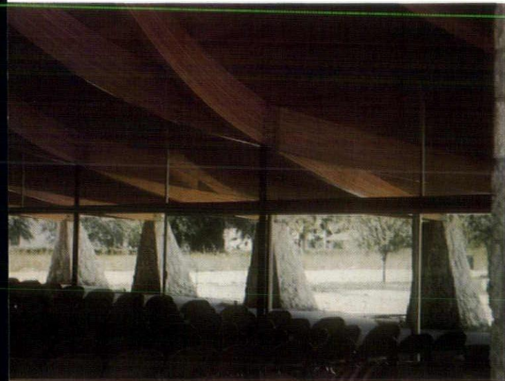
St. Paul's Lutheran Church in Sarasota was designed by Victor Lundy in 1958. This church uses laminated timbers to create wonderful three-dimensional sculptural surfaces.
