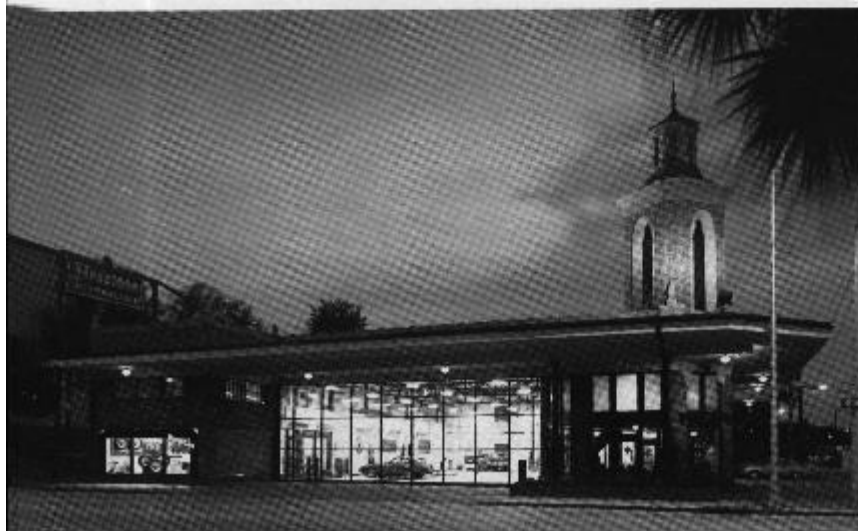
The Firestone Tire and Rubber Store in downtown Orlando. The building was restored by Leslie Divoll, AIA, of the Orlando architectural firm of Divoll and Yielding. Photo by Bob Braun.
