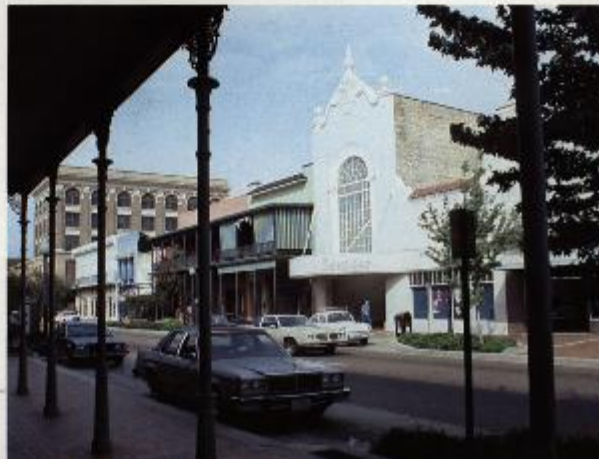
The restored Saenger Theatre is the center piece of Palafox Street, Pensacola's main downtown street. Palafox Street has been restored architecturally, but not yet commercially.
