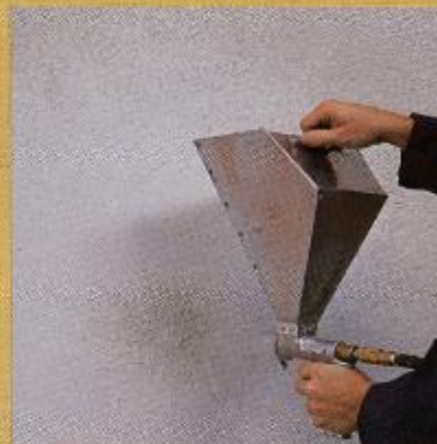
Finish coat is applied
