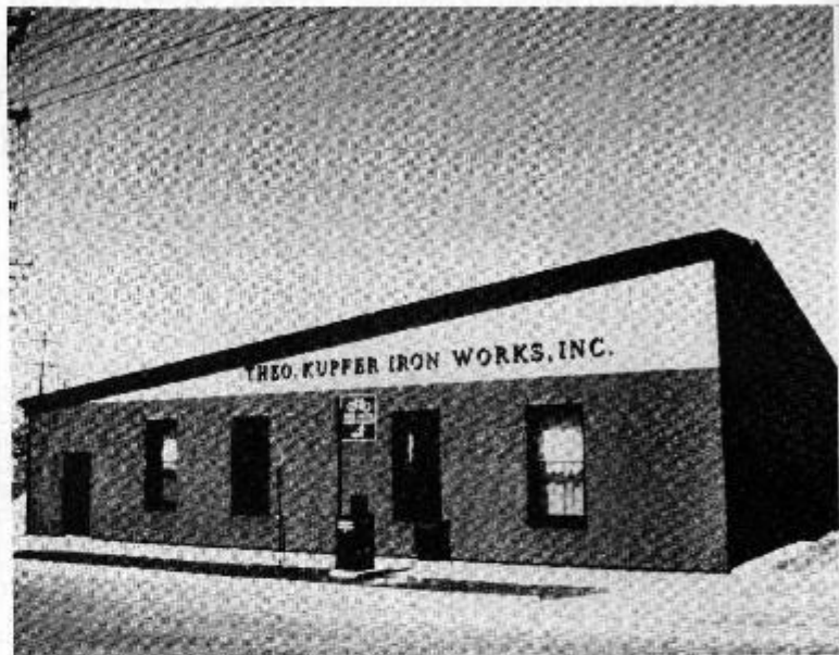
Above: A two-color exposed aggregate finish was selected to complete the exterior wall insulation system in the manufacturing facility renovation project. Photos courtesy of Dow Chemical Company.
