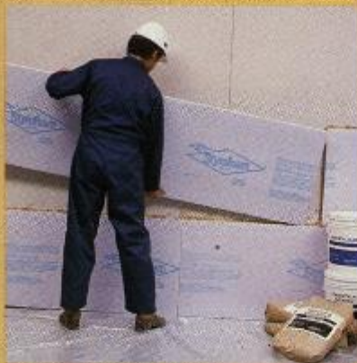
Boards of STYROFOAM brand insulation are set in place
