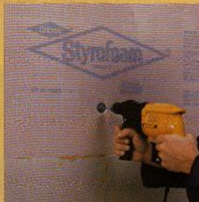
Fiberglass mesh is applied, mechanical anchors are attached
