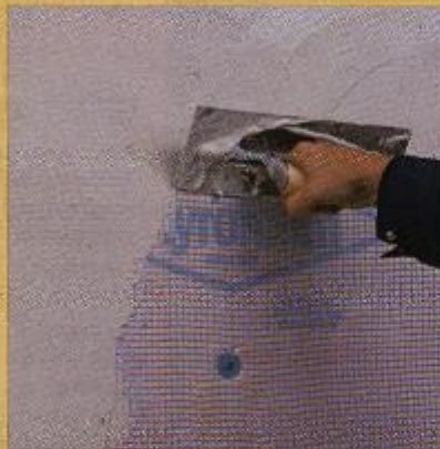
Base coat is applied with trowel
