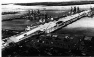
Pier Zulu, designed by Gee & Jenson of West Palm Beach, is the U.S. Navy's first double deck pier. Photo courtesy of Colee & Co.
