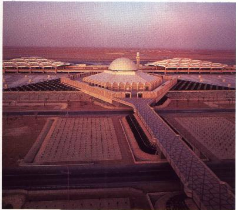
The centerpiece of King Khalid International Airport, the hexagonal Mosque is flanked by triangular terminal buildings having 30-60-degree angles. Not only are these angles basic to traditional Moslem design, but they also give aircraft the maximum maneuverability between buildings at the 70,000 acre airport. Photo by Gregory Murphy © 1984.
