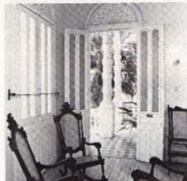
Porch and entry in San Germán house showing perforated wood transoms used for ventilation.
