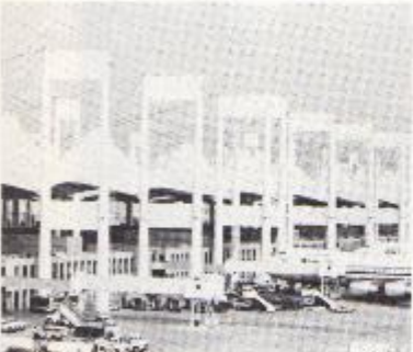
The Hajj Terminal at King Abdulaziz International Airport provides shade for the Moslem Pilgrims on route to Mecca. Design, fabrication and installation of the 5.5 million square feet of fabric roof was completed four months ahead of schedule. Photo courtesy of Owens-Corning Fiberglas
