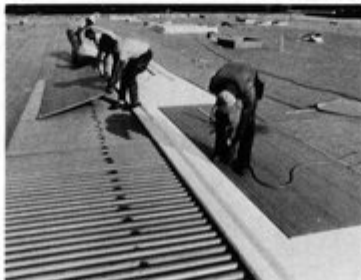
A total of 1.3 million board feet of EPS provided an insulation value of R-20 at Bay Area Outlet Mall, Tampa.
