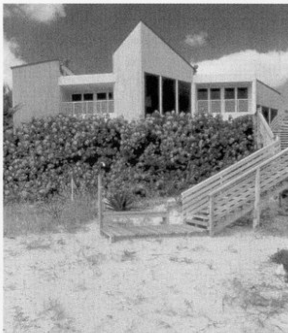
Only a ramped cedar footbridge arches above the sand dune's natural vegetation. The house was built up above the dune for best visibility and water protection and was designed for hurricane conditions.
