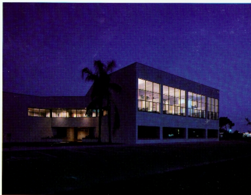
Top: Axonometric of reception area and below, exterior of building after dark.
