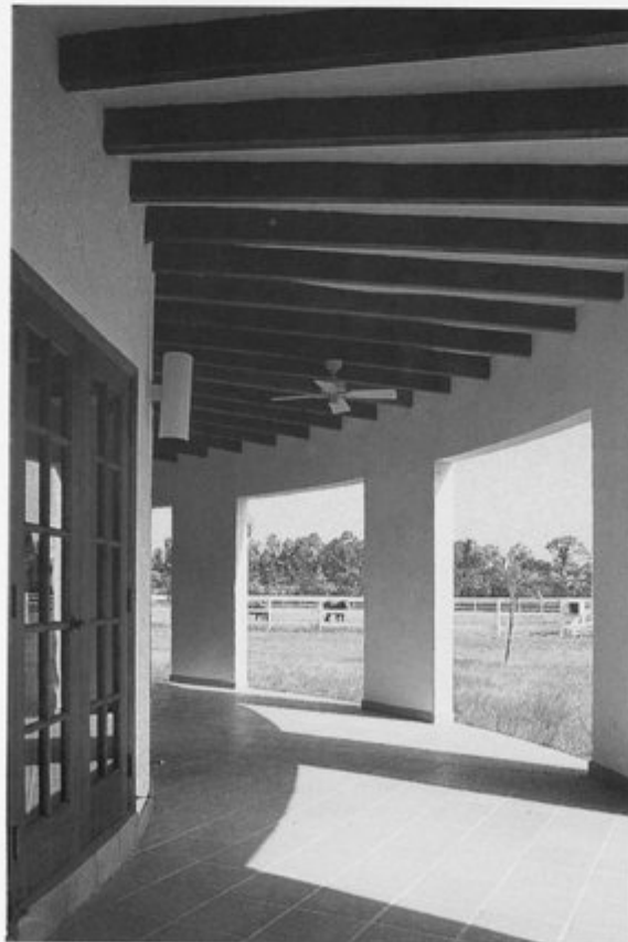
Top photo, West elevation and lower photo, porte cochere interior. Photos by Patti Fisher.
