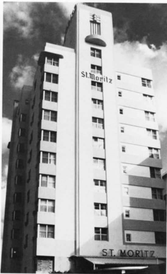
The 1939 St. Moritz Hotel in Miami Beach will undergo a restoration based on Sasaki Associates' schematic design.
