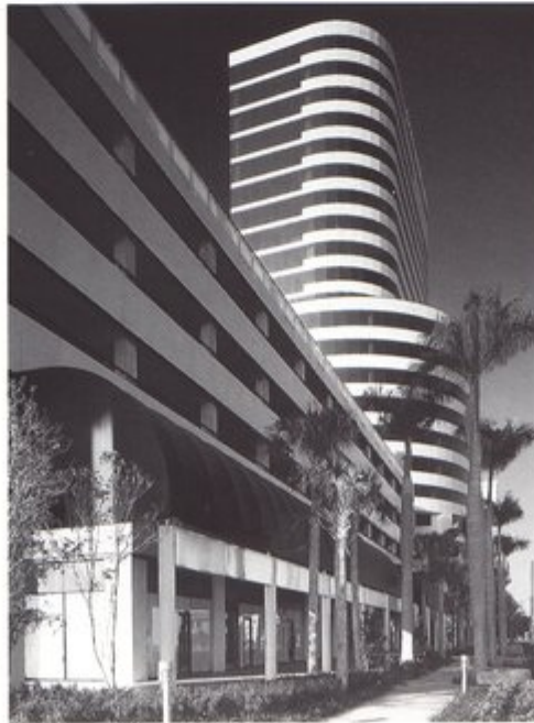
Opposite page, top; Federal Building-U.S. Courthouse by William Morgan Architects, P.A. Photo by Dan Forer. Bottom: The Broward County Main Library was a joint venture of Gaije Papachristou Smith, New York, and Miller & Meier & Associates, Fort Lauderdale. Photo by Steven Brooke. This page, top: City Park-Urban Plaza and Municipal Parking Garage designed by Donald Singer, FAIA. Photo © Wolfgang Hoyt Esto. Left: Broward Financial Center by the Nichols Partnership, Inc. Photo by Steven Brooke.
