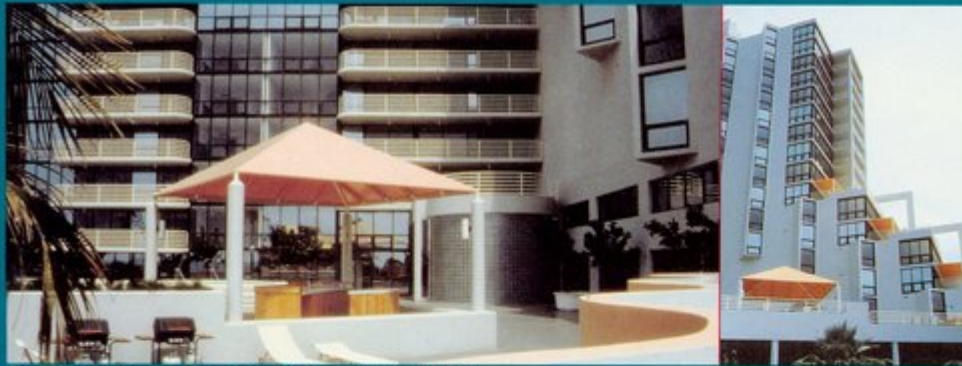
First Place, Multi-Family Residential, The Terraces, Naples, Florida
