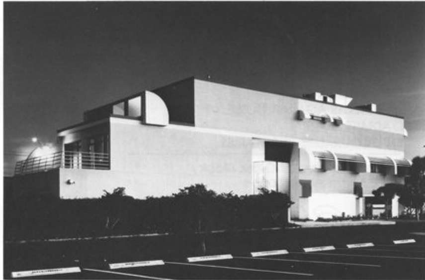
City of Fort Lauderdale Utilities Administration and Laboratory Facility by Miller Meier Kenyon Cooper Architects and Engineers, Inc.
