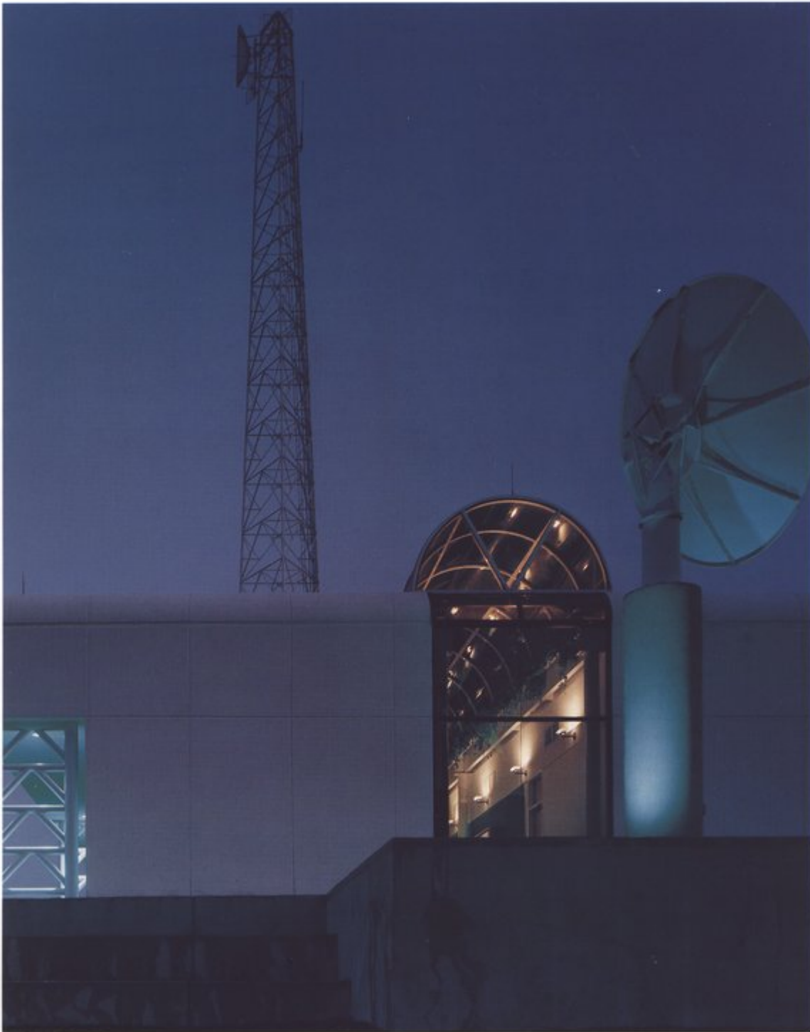
Opposite: The Peabody is one of Orlando's newest hotels. It was a project of The Nichols Partnership in joint venture with Vickrey Oversat Aesumb Assoc. Inc. Photo by Bob Braun. Above: Radio Station for WDBO/K92FM designed by Alexander W. Stone of Helman Hurley Charvat Peacock Architects, Inc. Photo by Esto Photographics, Inc.
