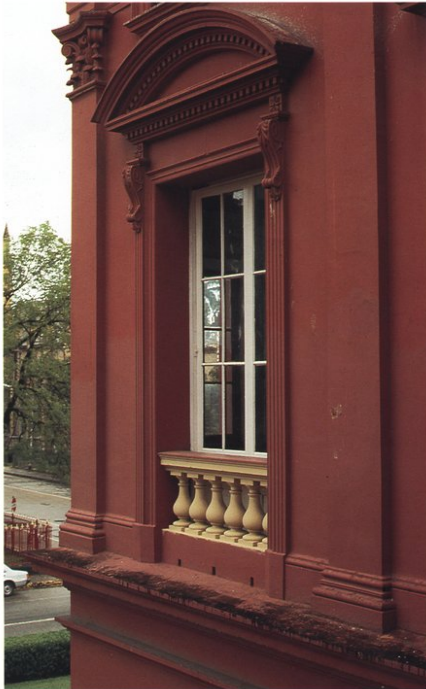
Window detail of Second Empire-style "Red House", Port-of-Spain's government center. The site developed by UF students is across the park in the background. Photo by D. Greer.
