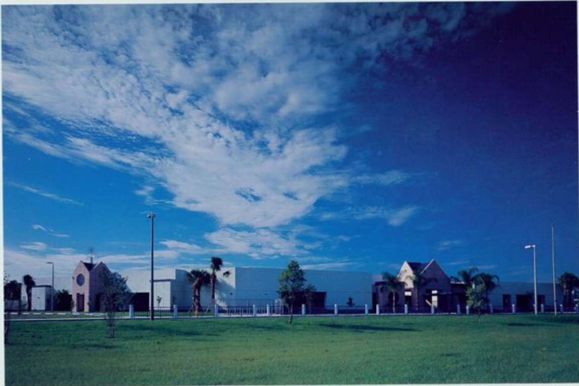
Pink porticos with royal blue pitched roofs draw the attention of students and visitors to important entry points. Photos by C. J. Walker.
