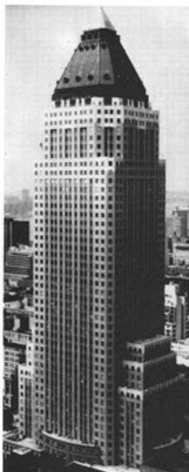
Worldwide Plaza in New York City was designed by David Childs of Skidmore Owings and Merrill's New York office. The construction of this 49-story office tower is the subject of a 5-part PBS film entitled "Skyscraper." Photo courtesy of WGBH Boston.
