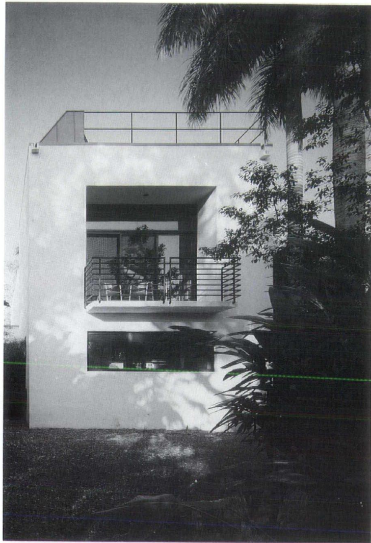
Photo, left, east elevation of office showing poured-in-place balcony and black metal railing. Photo by Steven Brooke Studios.
