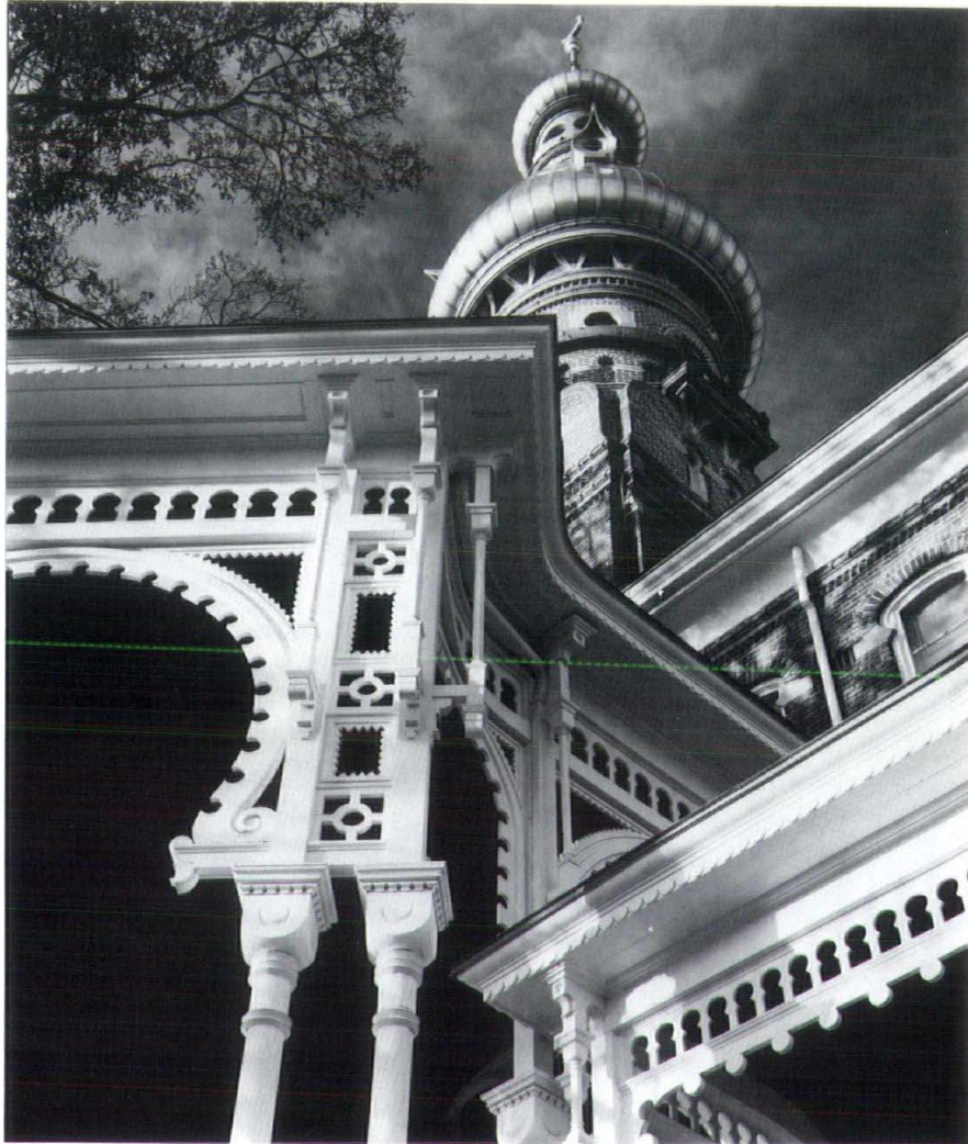
University of Tampa/Verandah Restoration Rowe Rados Hammer Russell Architects, Inc.
