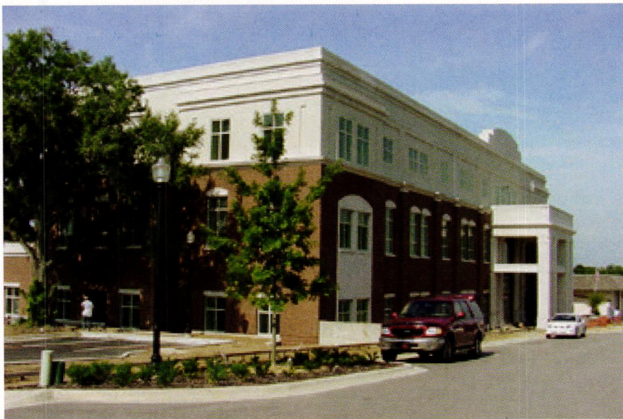
C.T. Hsu + Associates, P.A., is designer of the new Clermont City Hall, for which construction is now complete. The 32,000sf, brick and stucco structure is reminiscent of the architecture of Central Florida during the 1920s and was designed to be easily incorporated into the historical character of the existing downtown.
