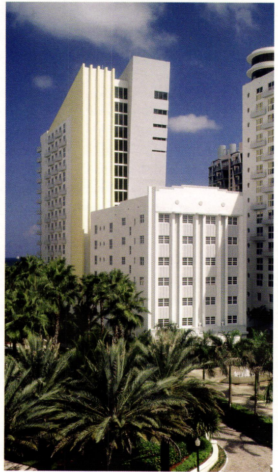
Photo, above: Collins Avenue elevation of the new resort complex. Facing page: the new Royal Palm Crowne Plaza Resort towers as seen from the ocean side. All photos by Steven Brooke.
