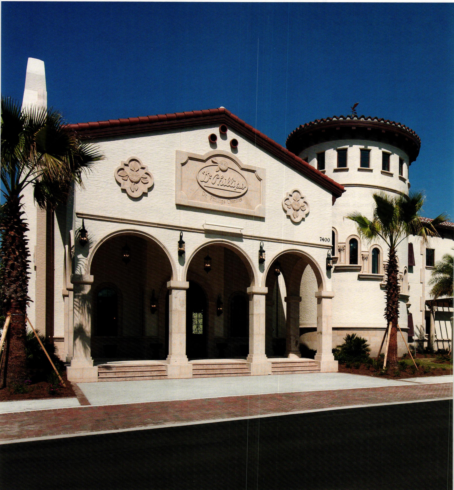
Partial view of the east elevation showing the main entrance. ALL PHOTOS BY BEN TANNER PHOTOGRAPHY, COURTESY OF SHENKELSHULTZ.
