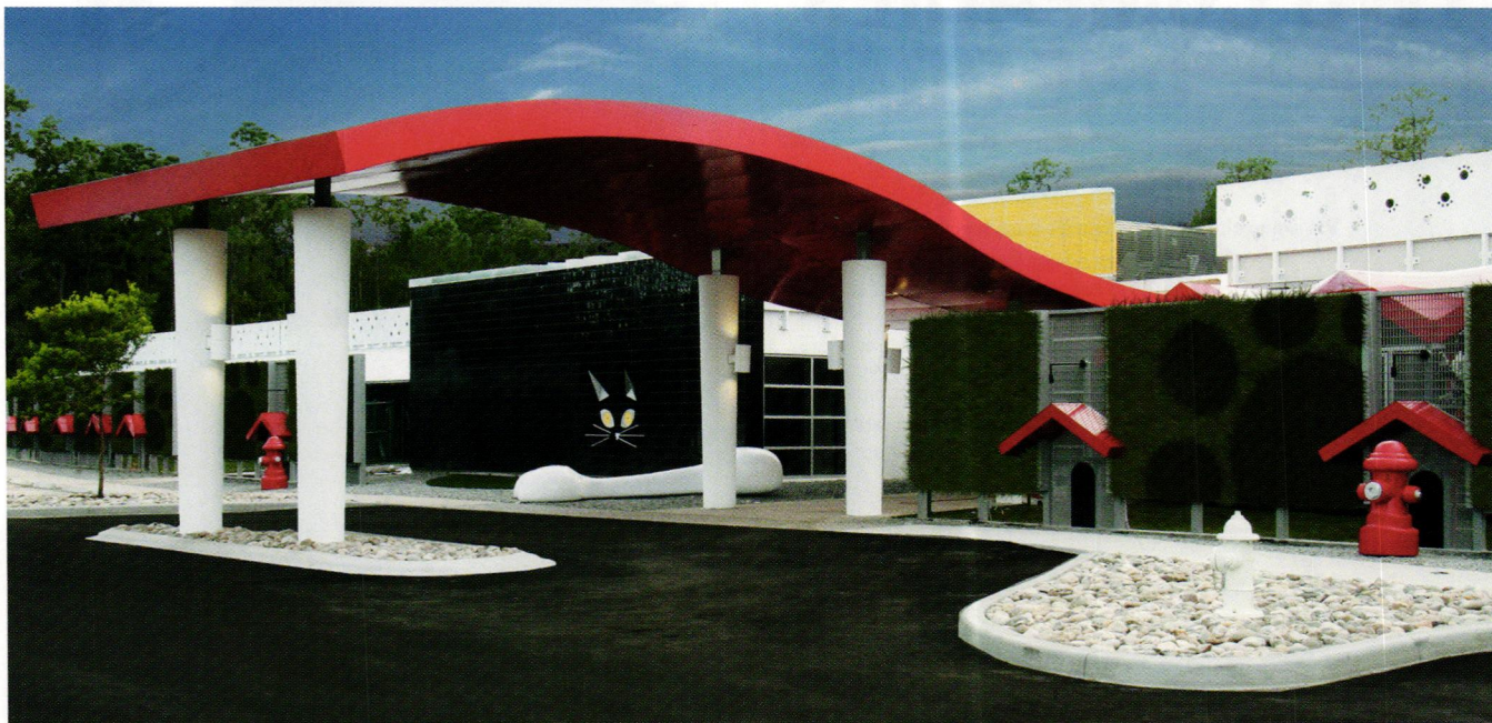
The main entrance to the hotel is beneath a covered walkway in the form of a tongue, a most familiar greeting image for pet owners. ALL PHOTOS BY RONEY MATEU, FAIA.
