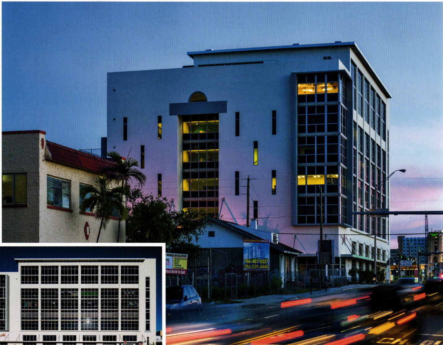
Evening view of the school from the southeast, top, and inset, east elevation with its huge expanses of glass allowing for panoramic views of the city.
