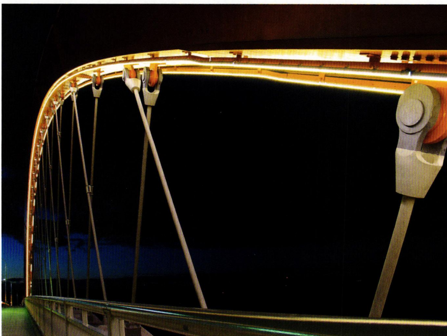
The bridges arch and cables looking down the shared-use railing.
