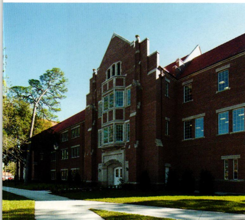
One of two entrances on the west side of the building. The architects used BIM software to reduce construction conflicts and improve inefficiencies.
