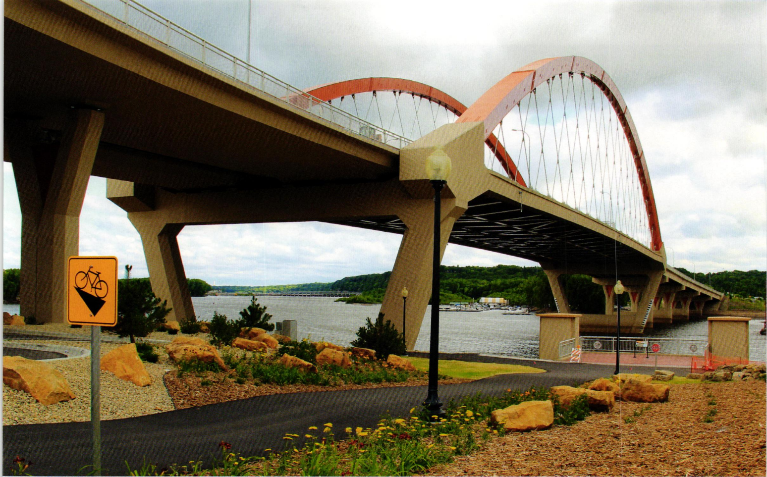
The new shared-use path showing the old bridge's piers repurposed into an overlook.
