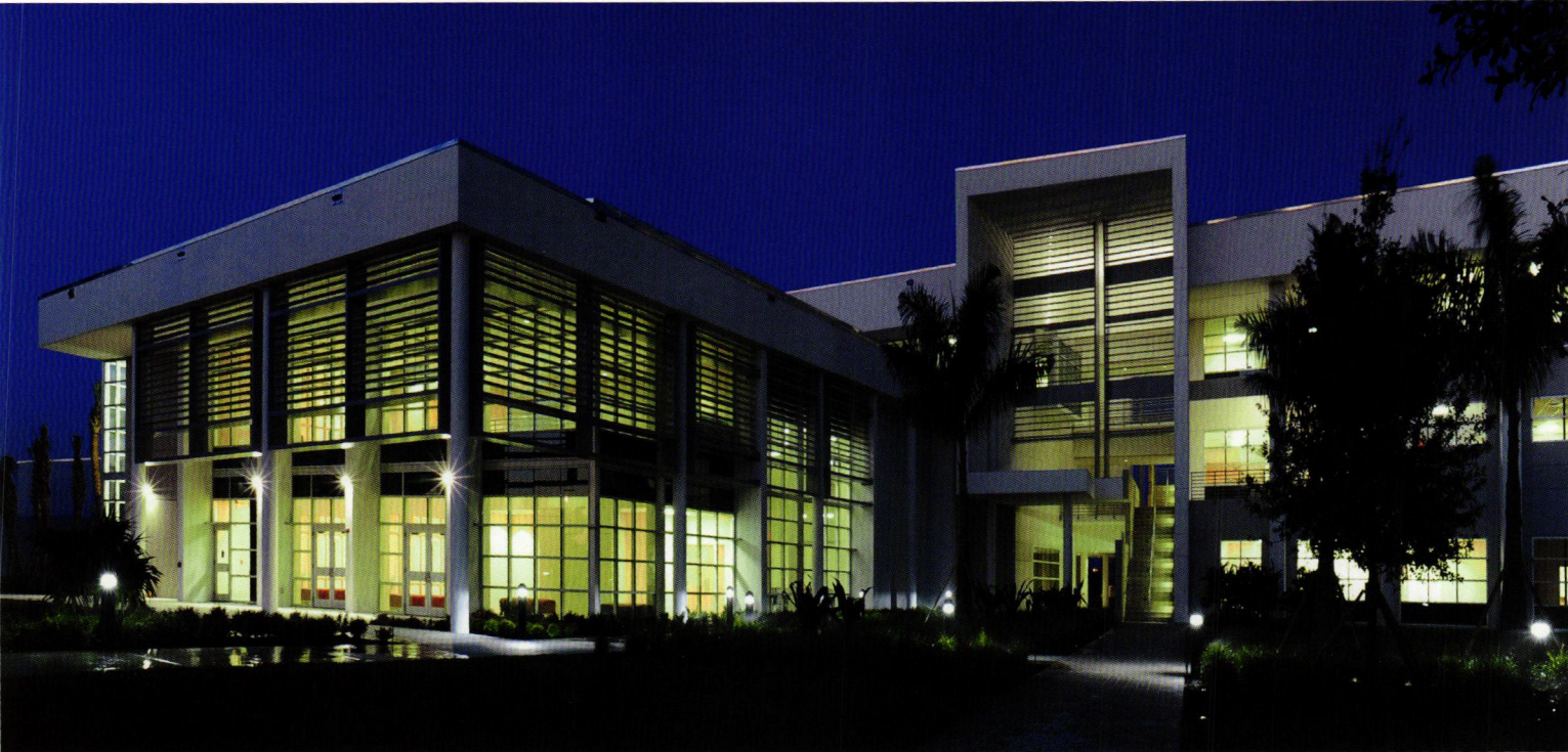
Above, main entrance to the training center at night showing the fully lit auditorium on the left. This entry leads directly into the "canyon," the main circulation area in the building. Below: Detail of the main entry.
