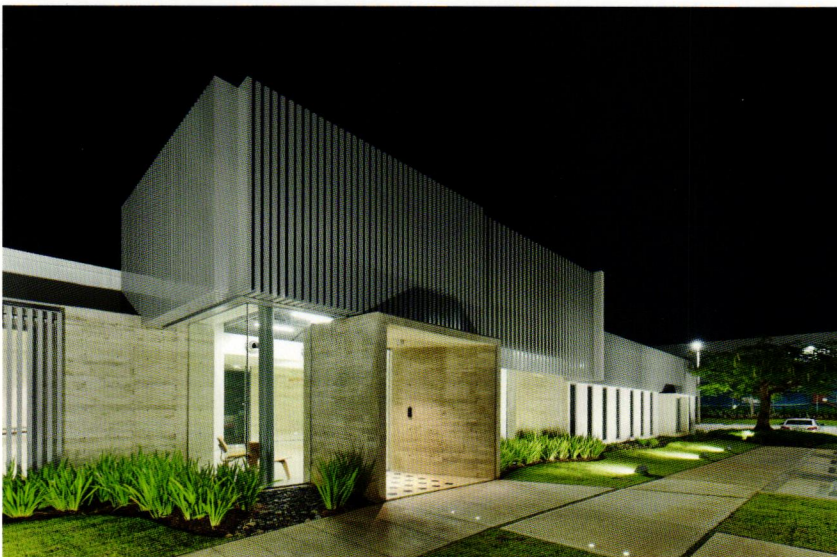
In this exterior view, some of the strategically placed alterations to the envelope can be seen.
