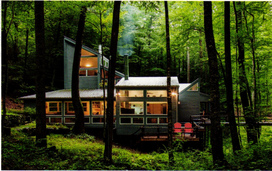
The house viewed from the south in a photo taken from the creek. New decks are visible as is the bridge from the house that crosses the creek.
