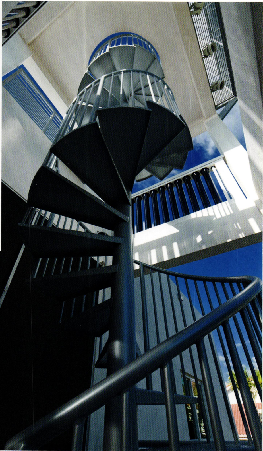
The 22-foot spiral stair extends up the tower from the loft level to the observation deck and incorporates 20 vertical solar hot water evacuation tubes sufficient to meet all user needs.
