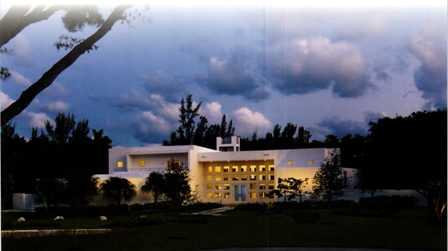
Front elevation shows minimal site disruption including a drivable grass surface in lieu of pavement. All photos, excluding aerial, are by Dan Forer.
