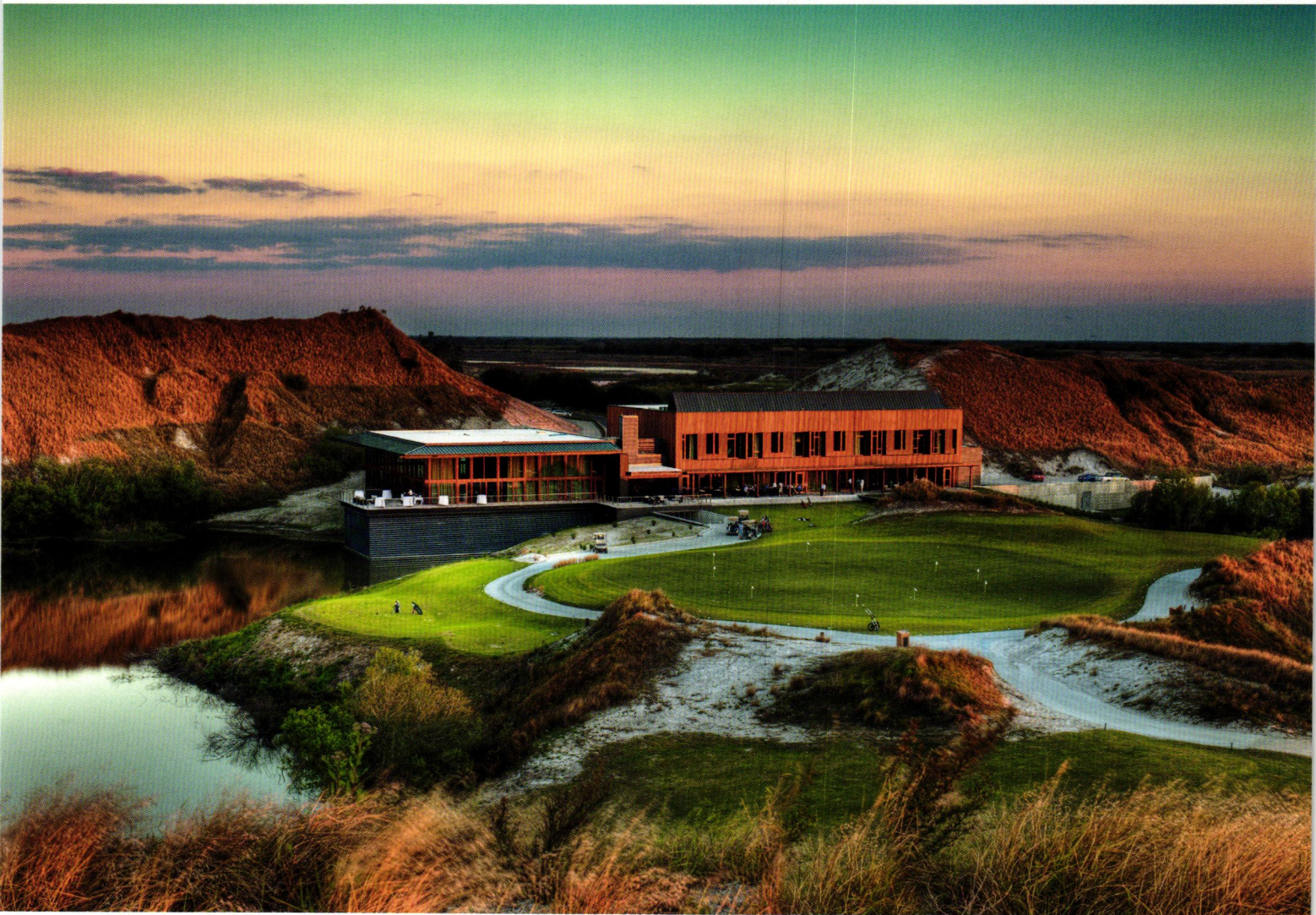
Streamsong Clubhouse viewed from the west.
