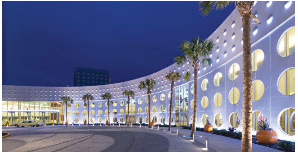
The entry court is connected to the double-height concourse by a curvilinear arrival building that is screened with perforated metal panels.
