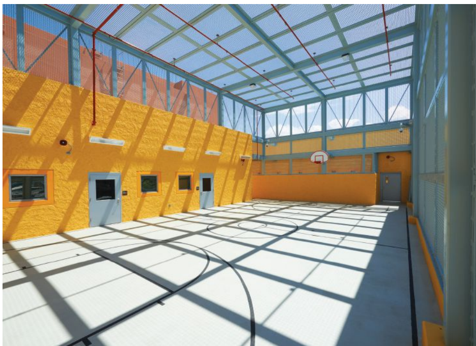
The third floor's central outdoor recreation area for inmates is located between housing units and features Tremco waterproof athletic surfacing on top of concrete floor.
