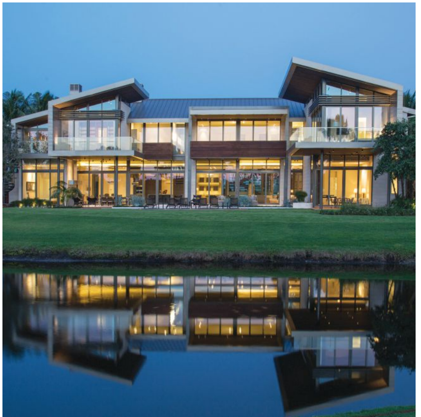
The rear façade at dusk.
