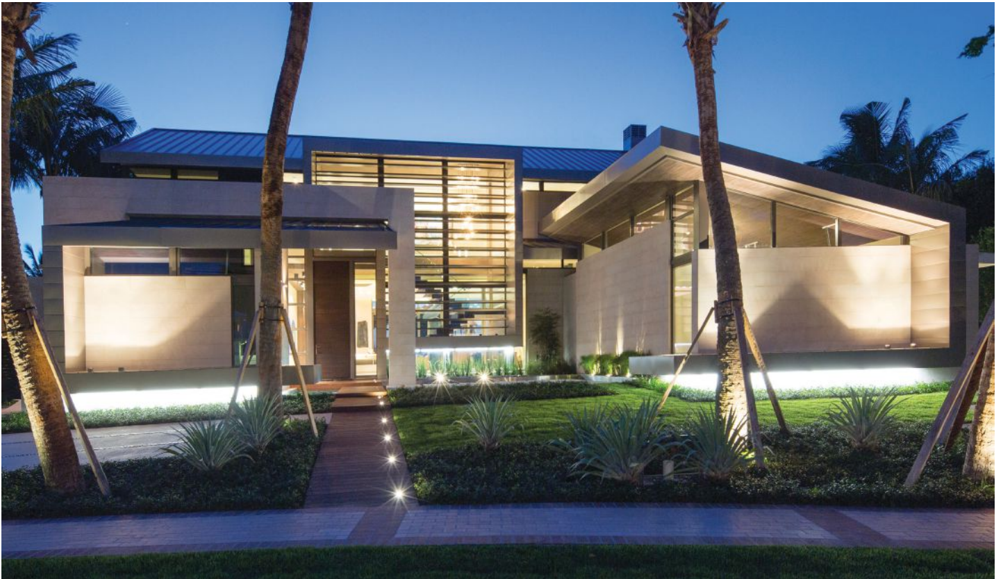
The front elevation is introverted with the two side pavilions designed to focus the visitor toward the entry. The large bay window is clad in metal frame, and it highlights the double-height gallery containing the stair. Louvers provide privacy from the street and modulate the sunlight.
