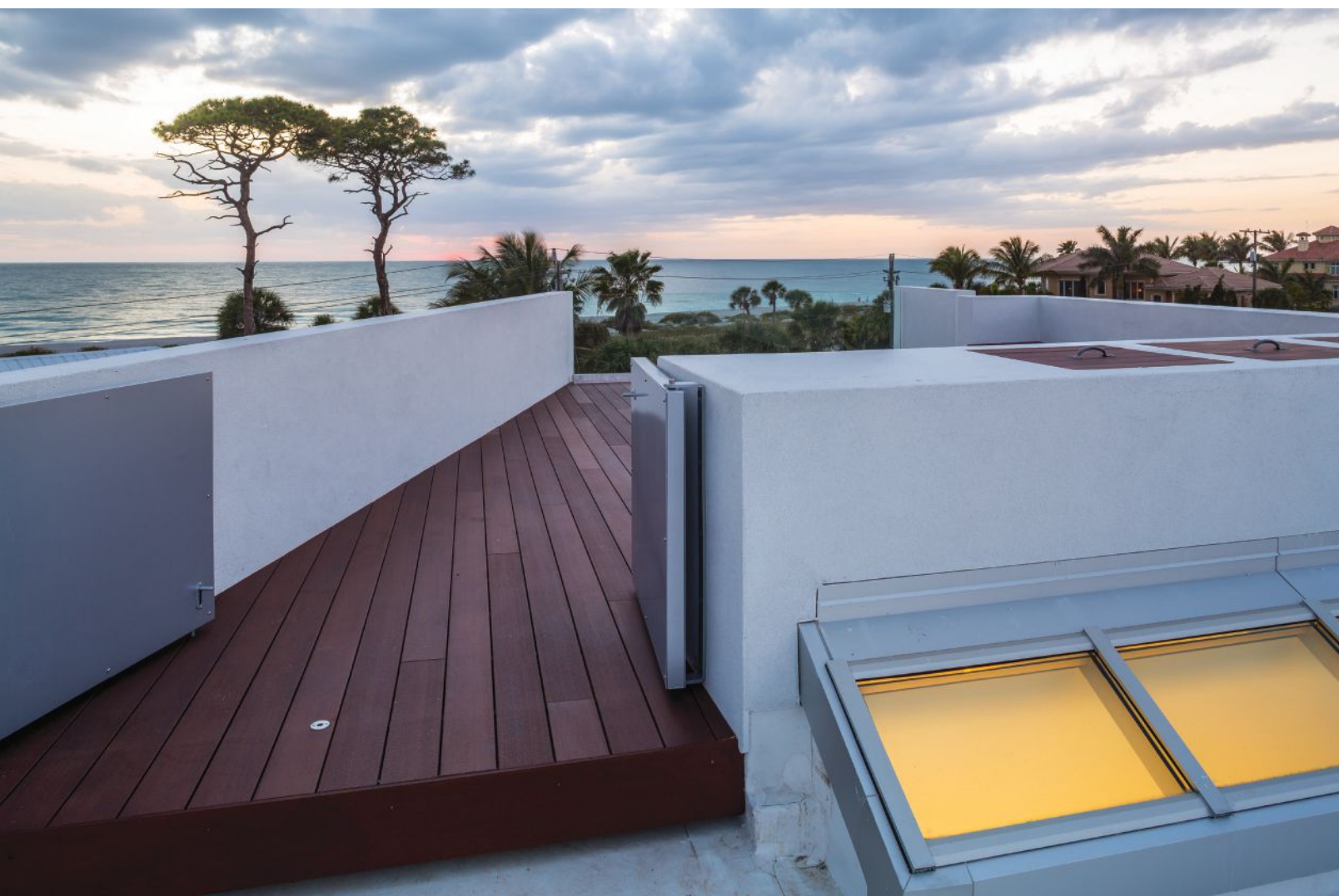
The roof terrace offers views of the Gulf of Mexico. A linear skylight brings daylight into the dining room below.
