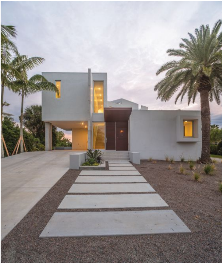
A two-story exposed concrete wall separates the pedestrian entry from the vehicular entry. The carport is raised to meet the required floor elevations of the house.
