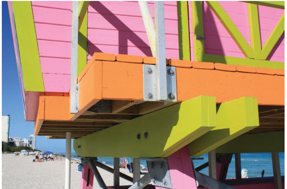
Tower detail showing underpinning, bolted cross-bracing and supports.
