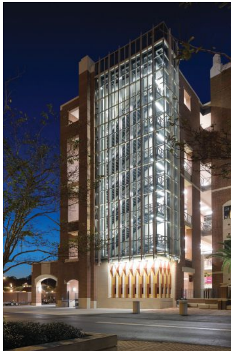
Night view of west circulation tower and the support framing for the curtain wall seen from inside the stair tower.
