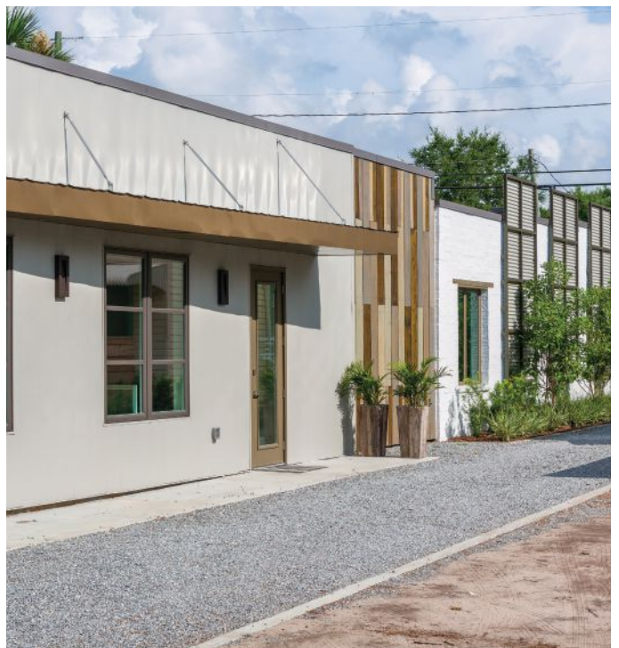
Exterior of building
