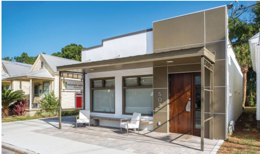
Main façade following renovation
