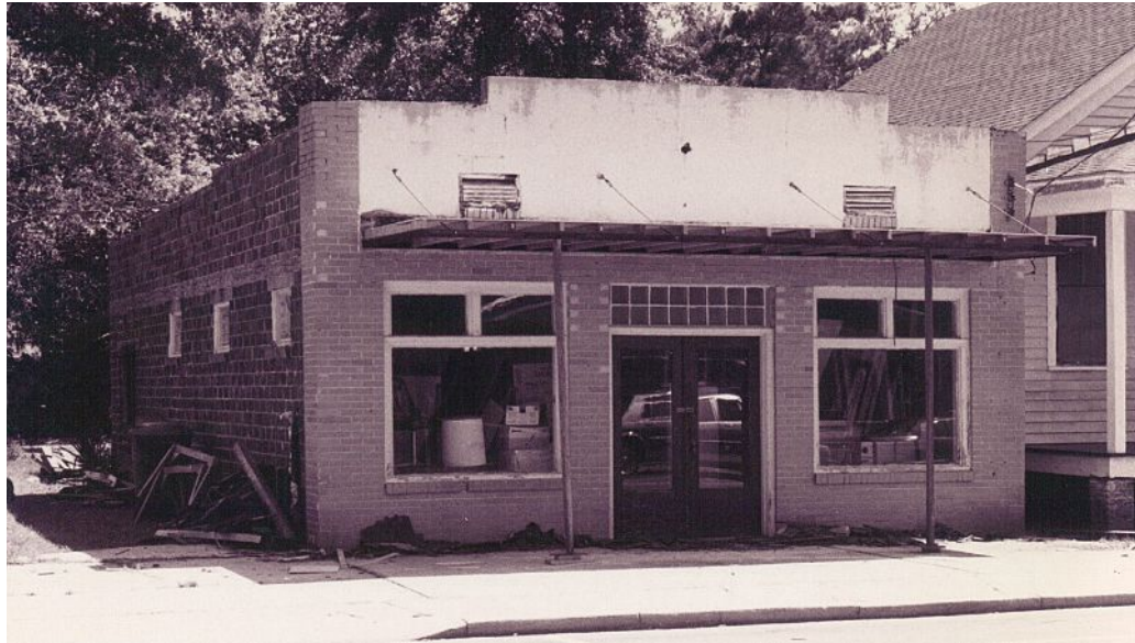
The historic grocery store prior to renovation
