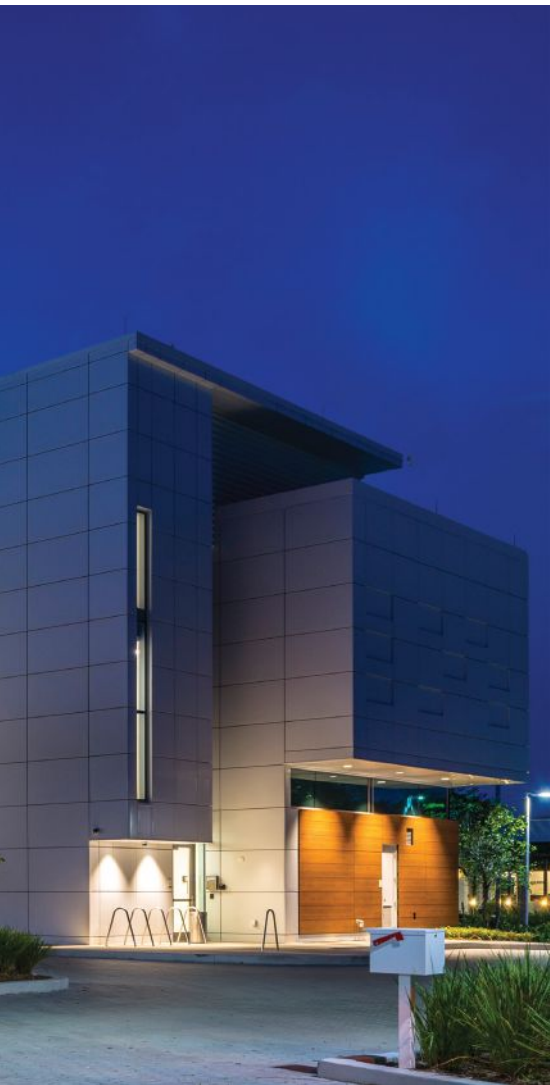
The finished structure shows how a complex, atypical design was implemented through use of available technology, teamwork and ingenuity. Left: The cantilevered second floor allowed for the creation of a sleek design with well-concealed complexities. Right: The incorporation of the second story into the plan also allowed for the creation of a covered patient drop-off.
