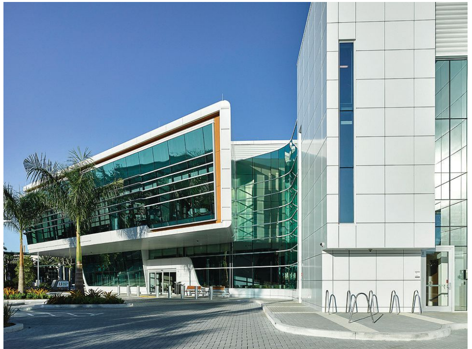
The finished structure shows how a complex, atypical design was implemented through use of available technology, teamwork and ingenuity. Left: The cantilevered second floor allowed for the creation of a sleek design with well-concealed complexities. Right: The incorporation of the second story into the plan also allowed for the creation of a covered patient drop-off.
