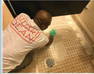
Grout & Tile Restoration – Revitalize Grout – Restroom Floors – Tenant Office Floors
