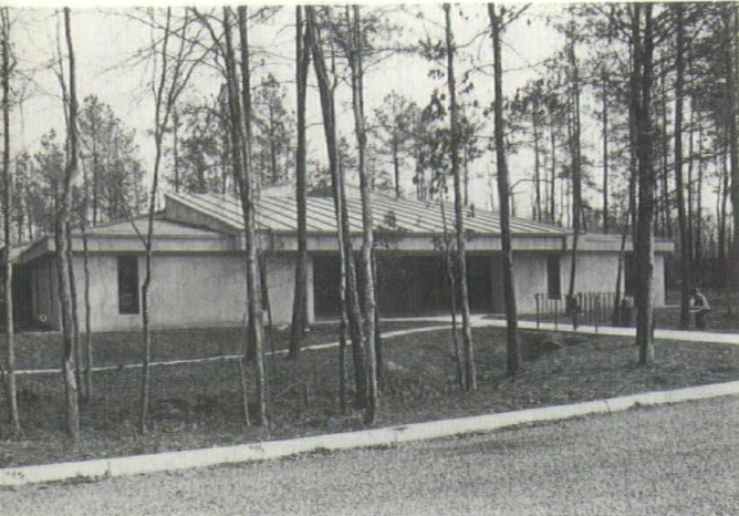
MERIT AWARD St. Bartholomew's Episcopal Church Architects: Highfill & Associates, Inc., Richmond, Va. Very good concern for program possibilities. Some question on entry to parking circulation. The exterior agrees with criteria, i.e., residential character. Some forced geometry.
