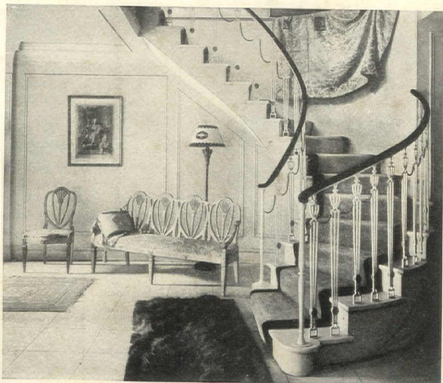
STAIRWAY IN MISS SWIFT'S BUILDING
