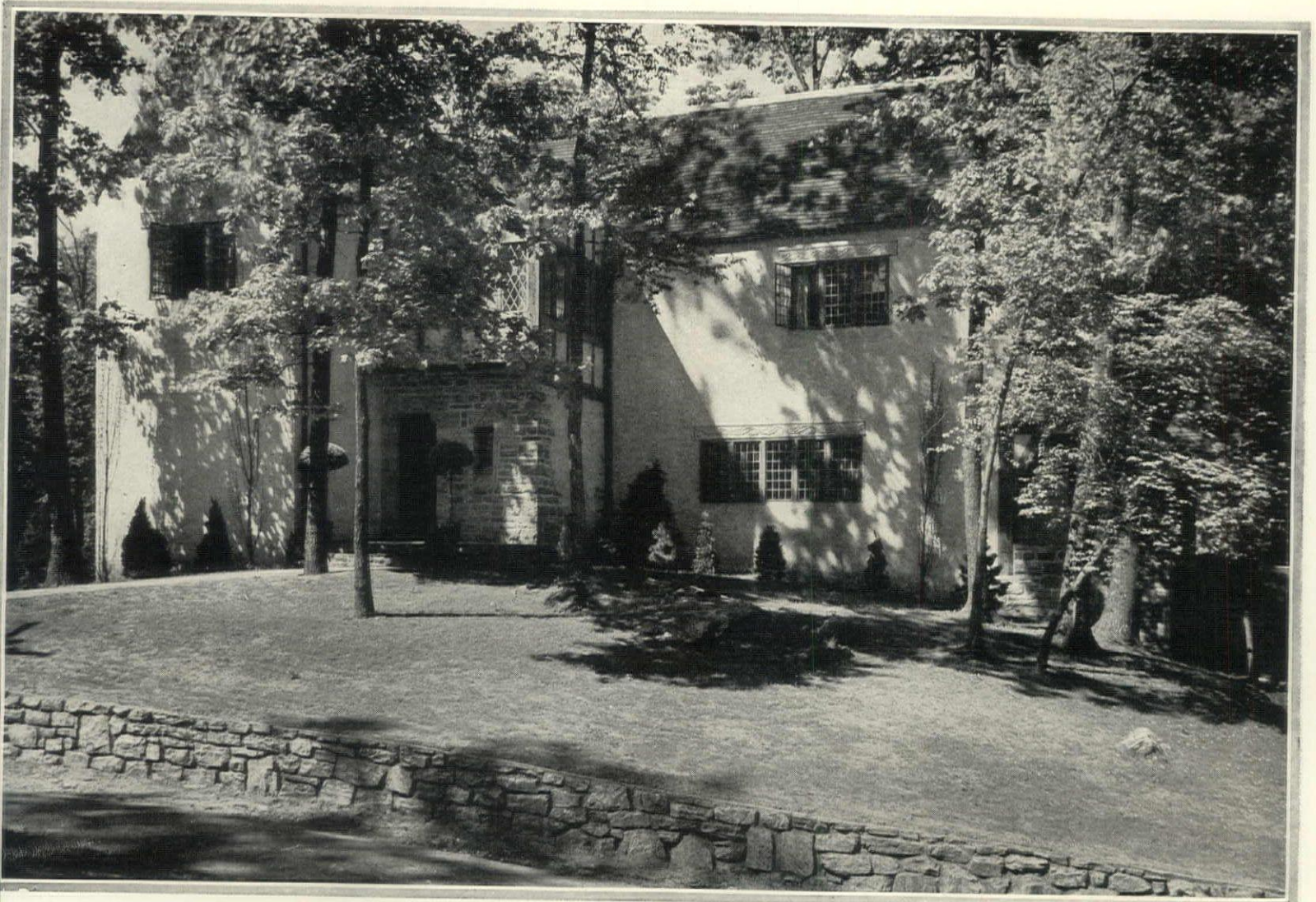
Not much is made of the entrance. It does not overshadow the house, as in many cases. It has been defined with fieldstone laid in wide bond and bled off into the stucco of the surrounding walls
