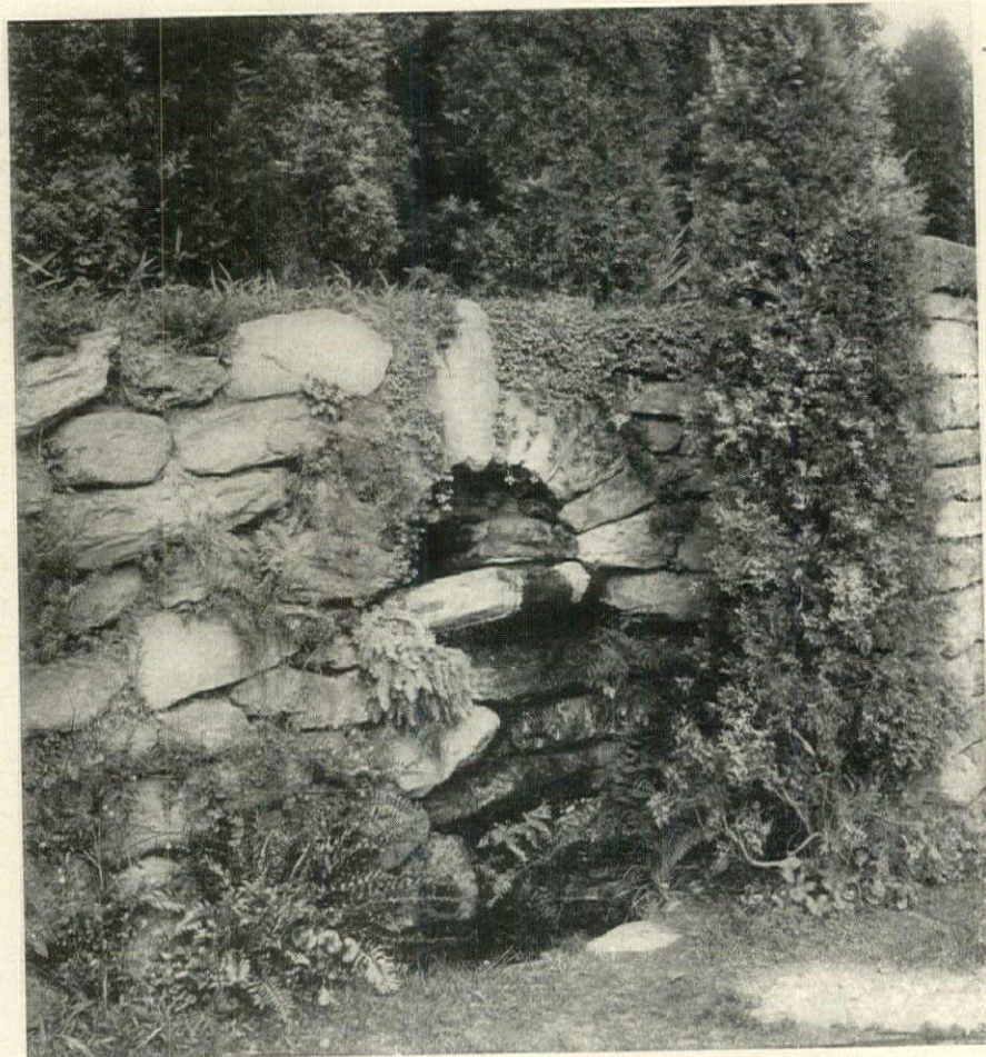
The ideal spot for a wall garden is a section of wall dry laid with sufficient space between the stones to allow for a little bed of loam in which the plants can take a grip
