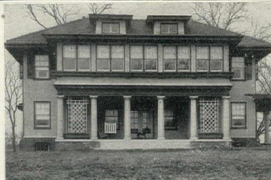
This is the General Manager's Residence of the wonderful R. A. Long farm, Longview, Mo. The buildings, all designed by Architect Henry S. Holt, Kansas City, Mo., have roofs of Imperial French Tile.
