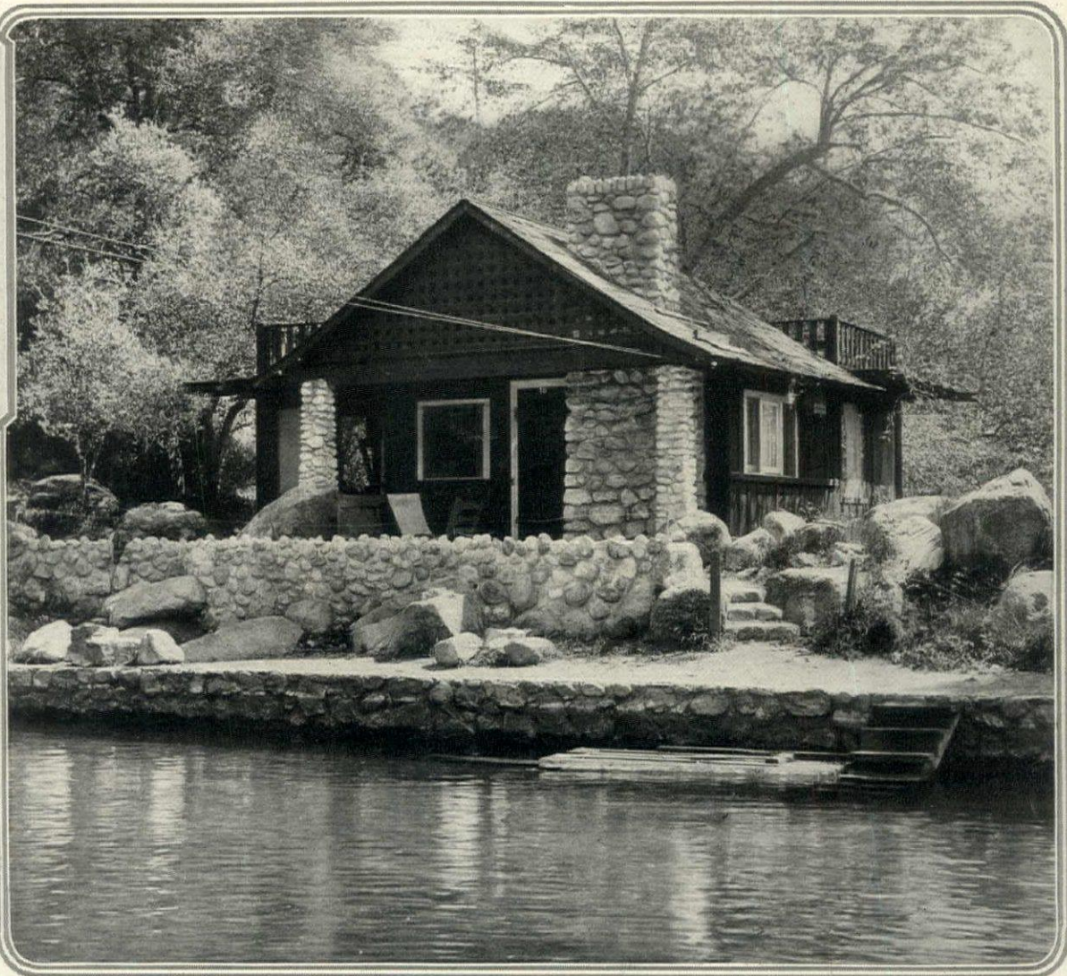
The outside walls are perpendicularly boarded and battened; the gables latticed and the roof shingled. Pillars and chimney are cobblestone. A cement-floored porch extends across the front. The cabin contains a combined living room and dining room, a bedroom, a sleeping porch and a small kitchen. Floors and woodwork in pine, finished in weathered oak stain in living room and white in bedroom. Approximate cost, $500. H. Whiteley, architect
