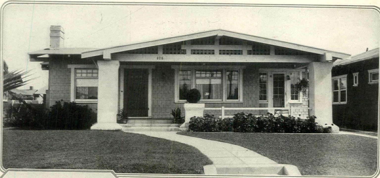
A popular type of California bungalow, suitable for a seashore cottage. Shingled asbestos roof, concrete pillars and porch floor. The plan shows the disposition of the rooms. Approximate cost, $2,350. E. E. Sweet, architect
