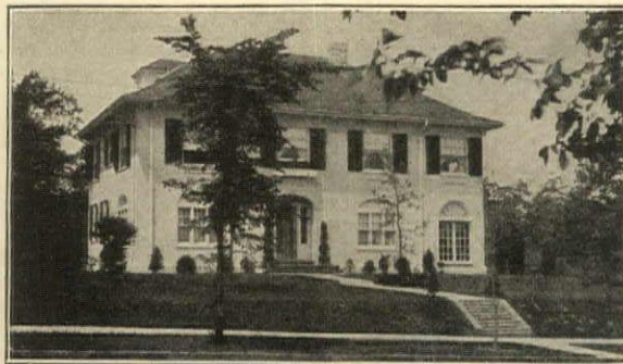
Kelsey Health Heated residence of W. J. Moffat, Edgehill Road, New Haven, Conn. Brown & Von Beren, Architects.
