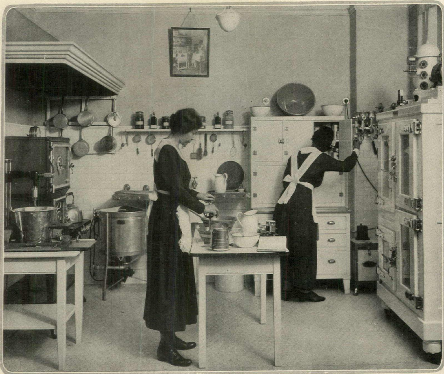
Almost everything runs by electricity in this elaborate kitchenette—electric stove, dishwasher, bread mixer, and ice machine. There are no back-breaking cupboard doors, but the utensils are hung up at a reachable height. Courtesy of the Edison Co.
