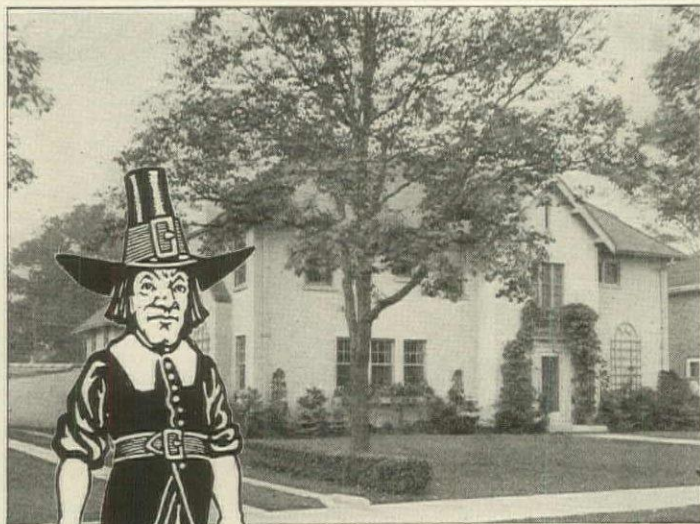
Residence of J. B. Book 385 Burns Avenue, Detroit, Mich. J. G. Steffens, Architect
