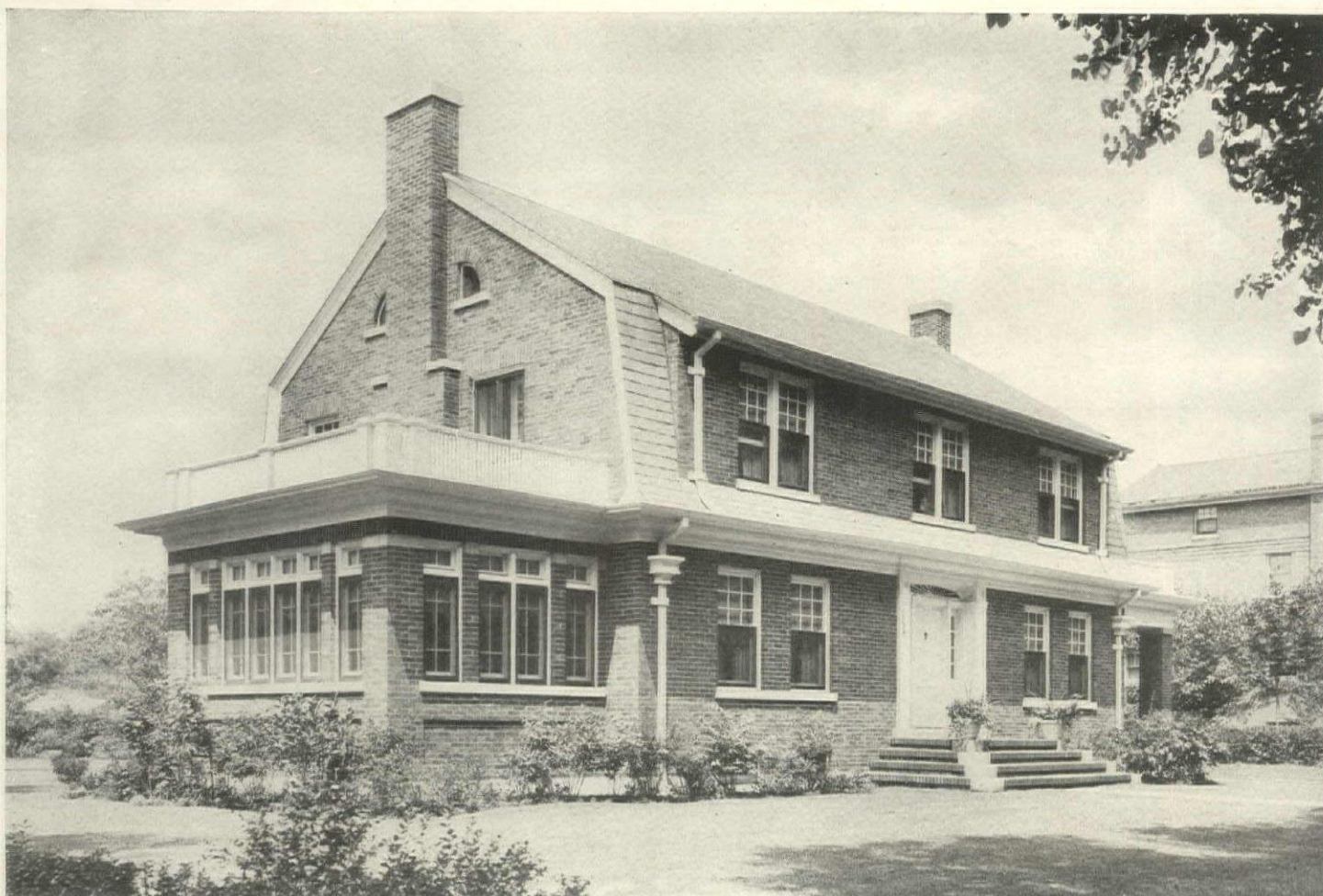
House at Chicago. Paul F. Olsen, Architect
