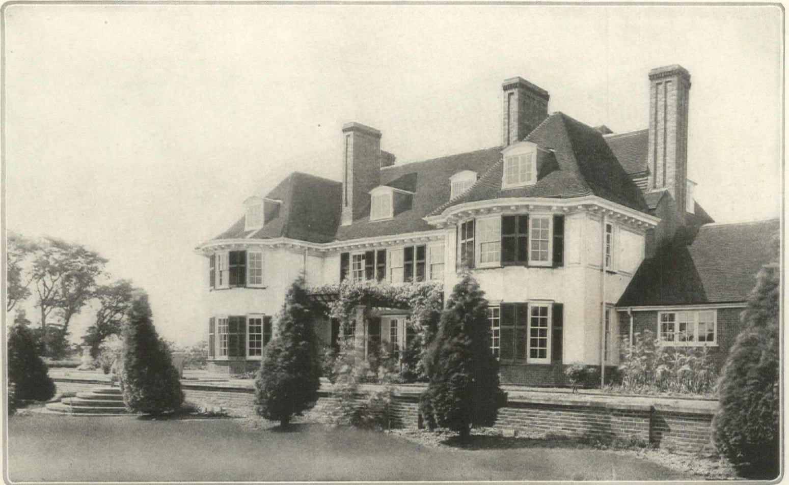
Green Heys, the residence of G. H. Garrett, at Snape, Suffolk, England, is a modern house built in the Queen Anne style, but following the Suffolk tradition in the detail of the plaster work. The relative proportions of the Queen Anne type are retained while the quasi-grandiose effect generally associated with Queen Anne architecture is avoided in adapting this classic model to modern requirements
