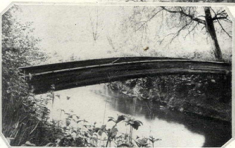
A foot-bridge made by fixing between blocks on either bank two boards slightly longer than the distance between blocks, causing an upward bend; then laying on other boards and bolting them
