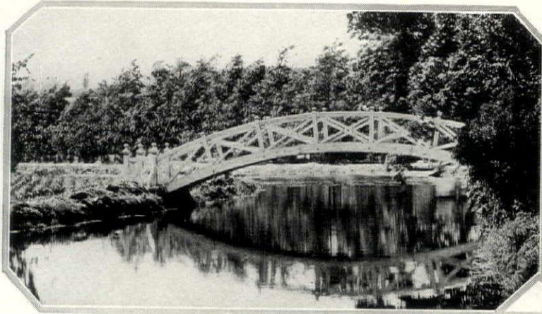
Built in sections clamped together with iron bolts, this single span wooden bridge, with the uprights of its balustrades radiating with the curve of the bridge, is reminiscent of Japanese work
