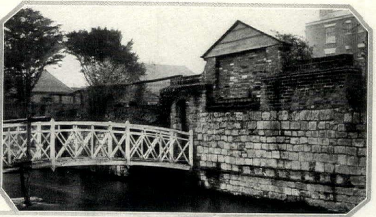
This wooden foot-bridge with its slightly curving span, built in three sections and bolted together, gives access from a house in the town to its garden on the other side of the dividing stream
