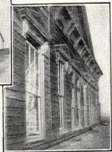
Catholic school erected at Alton, Cal., in 1870 now being torn down for its sound Redwood lumber.
