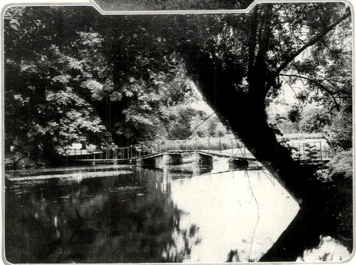
This causeway, with its simple rails and primitive planking, is supported on stone piers and rises in mid-stream to allow of the passage of boats. Its design is singularly appropriate to the scene's tranquillity
