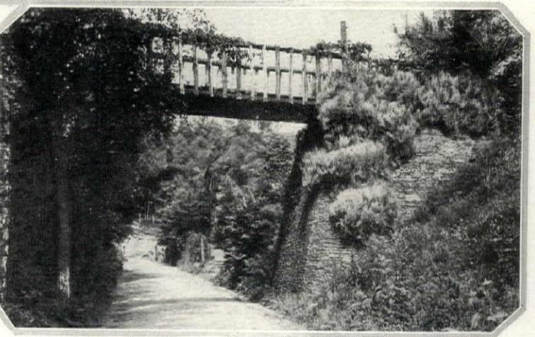
This drive to a country house is spanned by a straight wooden foot-bridge of rustic design. It is supported on one side by a dry-built stone bastion whose masonry bulk is masked in santolina
