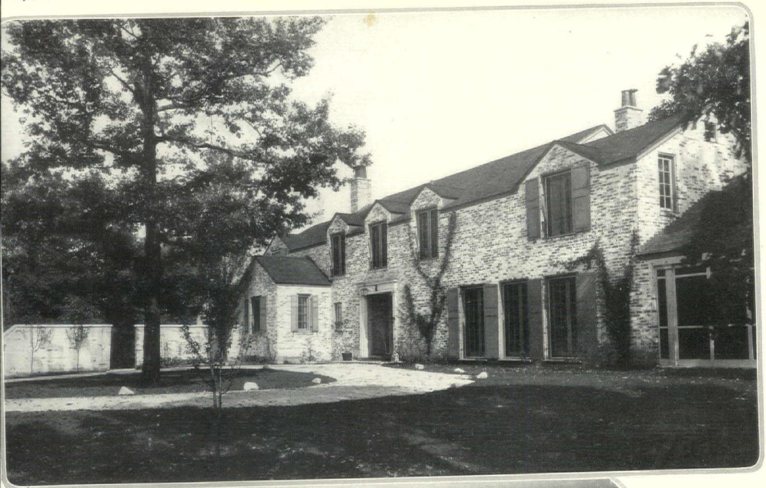
Dormers that break the line of the eaves and ranges of long French windows are Gallic details which were transported to this Illinois site. This is the entrance front
