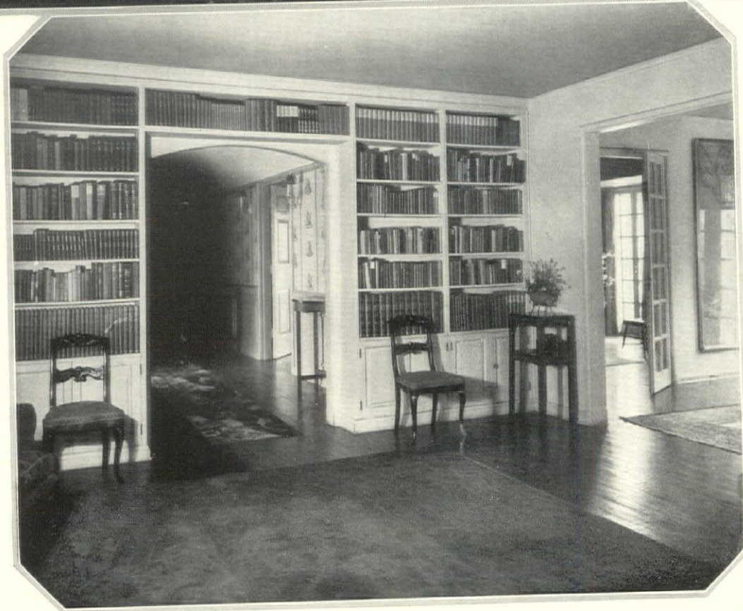
The library and its adjacent rooms are connected by wide openings more typical of American houses than French. The book-linteled doorway is a feature
