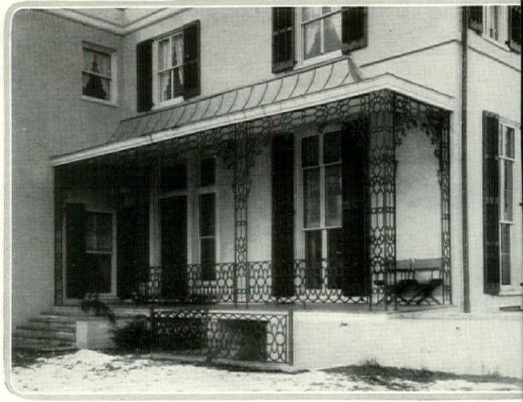
Cast iron verandah supports and balustrades have great silhouette value. They deserve a light background—a light toned stucco wall, or white-painted wood or brick
