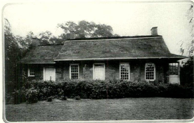
The farmstead shown on page 112 gave the lines to the garage. Its windows and doors were all taken from the old house without alteration or repairs
