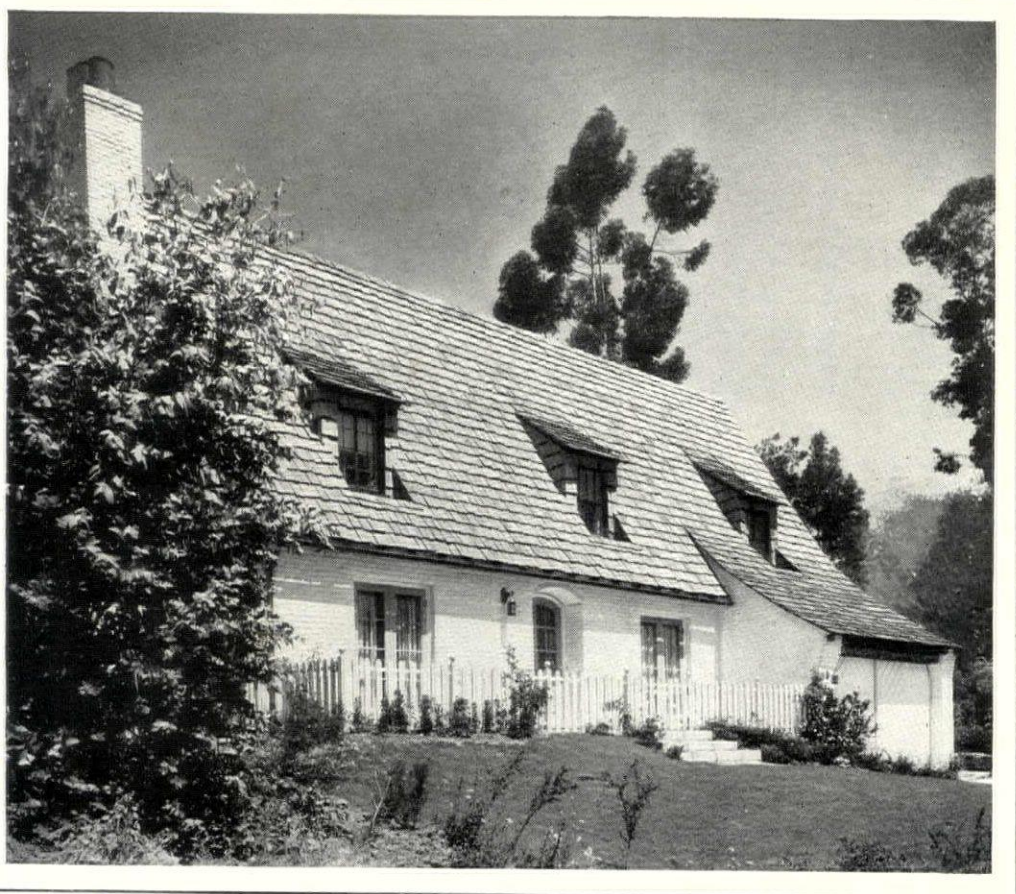
ARCHITECT FREDERICK H. REIMERS CHOSE CREO-DIPT HAND-SPLIT PILGRIMS TO GIVE THE ROUGH, RAGGED EFFECT HE WANTED ON THE ROOF OF THIS PIEDMONT, CALIFORNIA, HOME. ON THE SIDE-WALLS, FOR A PERMANENT, SOFT, FLAT WHITE EFFECT, HE USED CREO-DIPT DIXIE WHITE.
