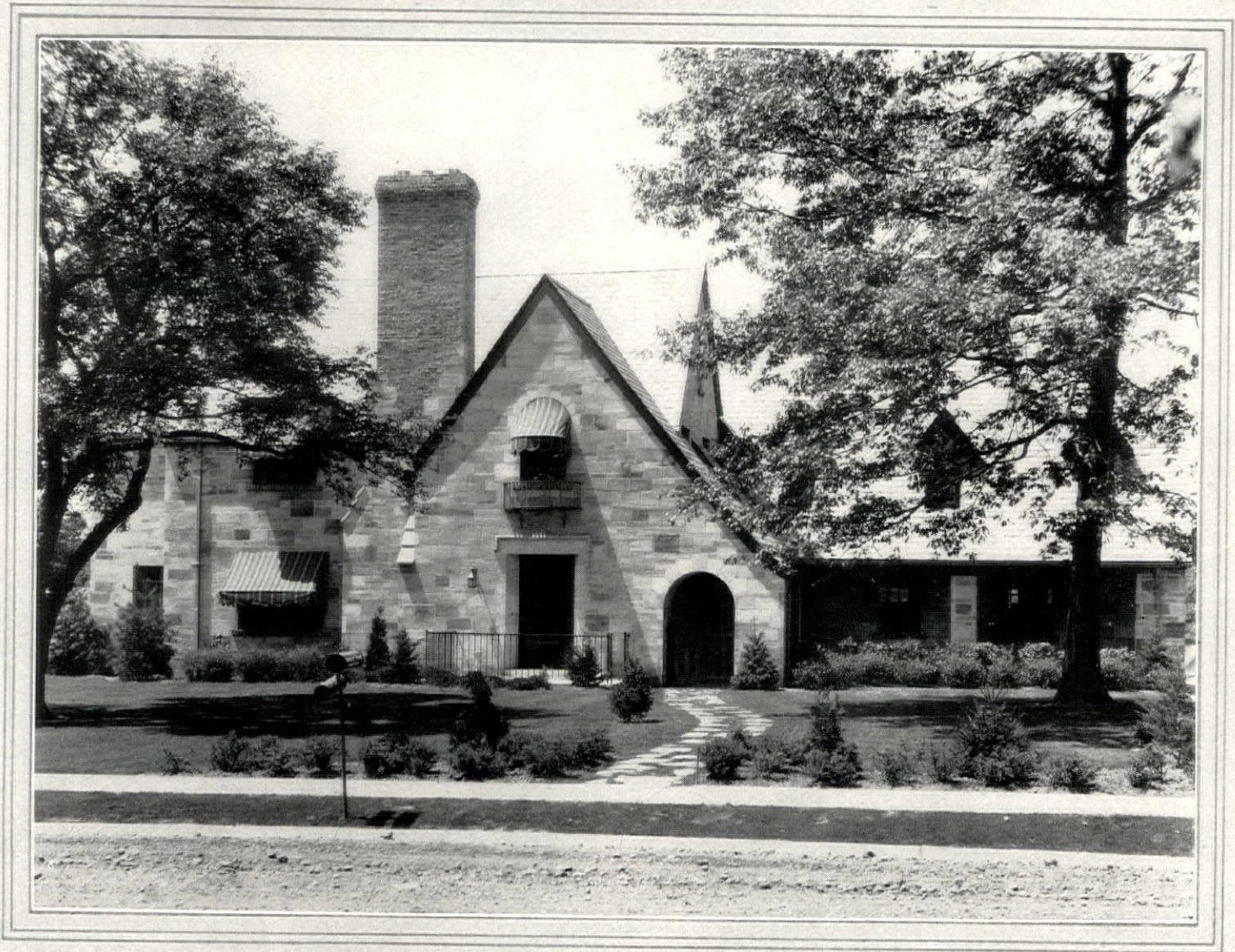
Residence, Birmingham, Michigan. A. L. Weeks, Architect. J. K. Burns, Builder. Old Gothic Shot-sawed Indiana Limestone.
