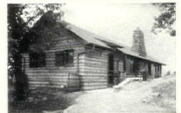
Cabot's Creosote Stain for added beauty and longer life of Shevlin Pine Log Siding. Architects, Magney & Tusler, Inc., Minneapolis.
