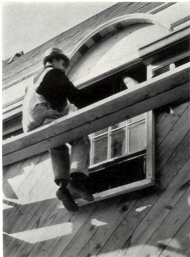
New materials and equipment, like these double-hung metal sash, were used
