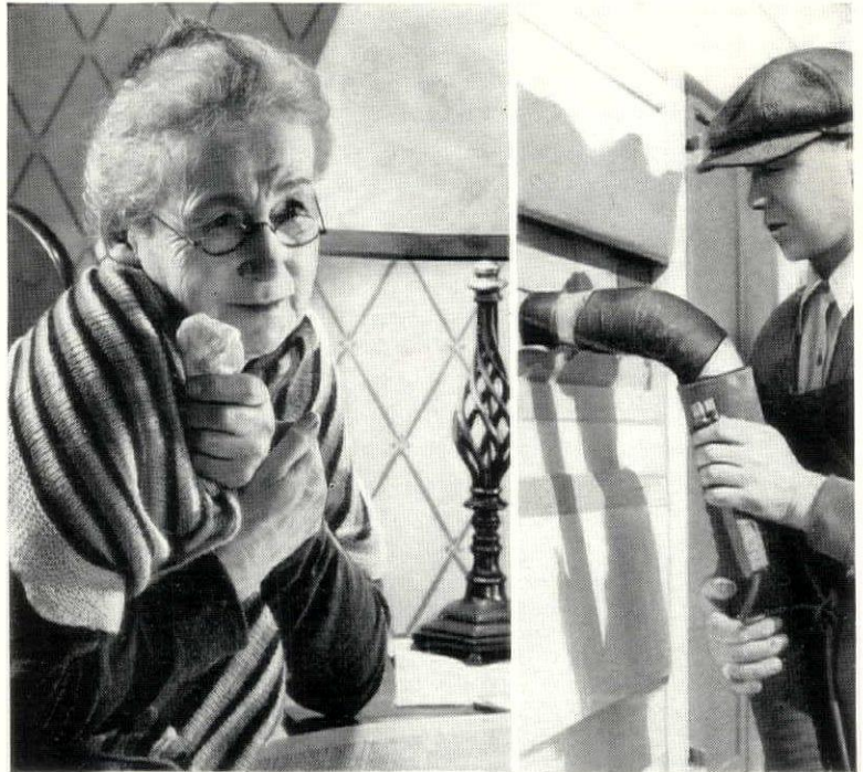
BY BLOWING J-M ROCK WOOL between attic floor joists and into hollow walls, this man puts an end to cold, draughty rooms.
