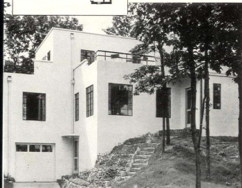
Modern home at Long Beach, Indiana—concrete walls, floors and roof decks
