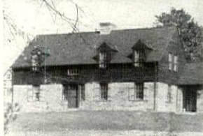
House at Hampton Park, Mo. Stained with Cabot's Stains. Architect, Angelo Corrubia.
