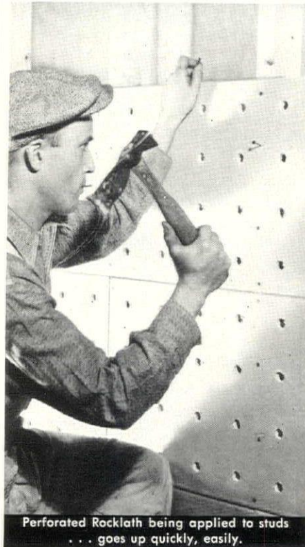
Plaster penetrates holes . . . gets strong grip on lath.
