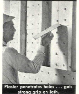
Red Top Plaster being applied to Perforated Rocklath.
