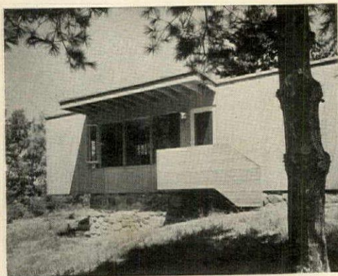
A roof overhang shades the living room window.
