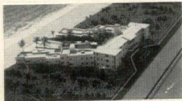
Lago Mar Hotel—Apartments
